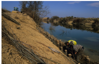
Photo 1: Engineering works along the river Vidourle (France)
