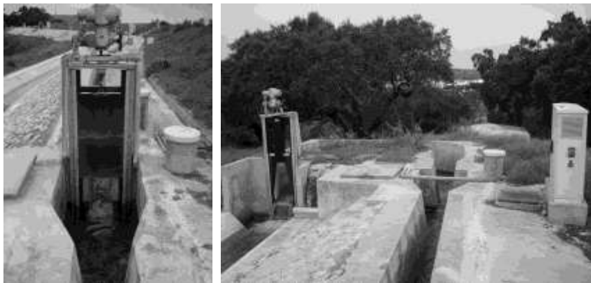
Figure 1. Two of the gates of the pilot canal used in the experiments.
