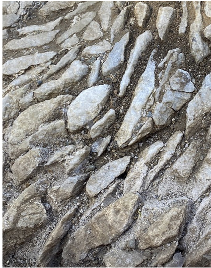
Fig. 3. Close-up of the marble-chip pavement of the Hall of Choral Dancers, likely a second use of construction waste generated by the project itself (photo by the author).
