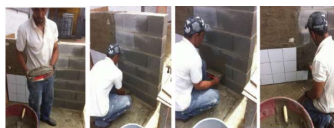
Figure 4 Images of applying the materials obtained from the tailings: a) in natura and b) calcined
