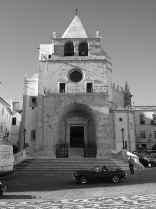
Fig. 27 The main façade after the conservation and restoration works of the historical mortars.
