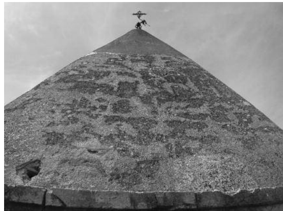
Fig. 4 Detail of the initial state of conservation.
