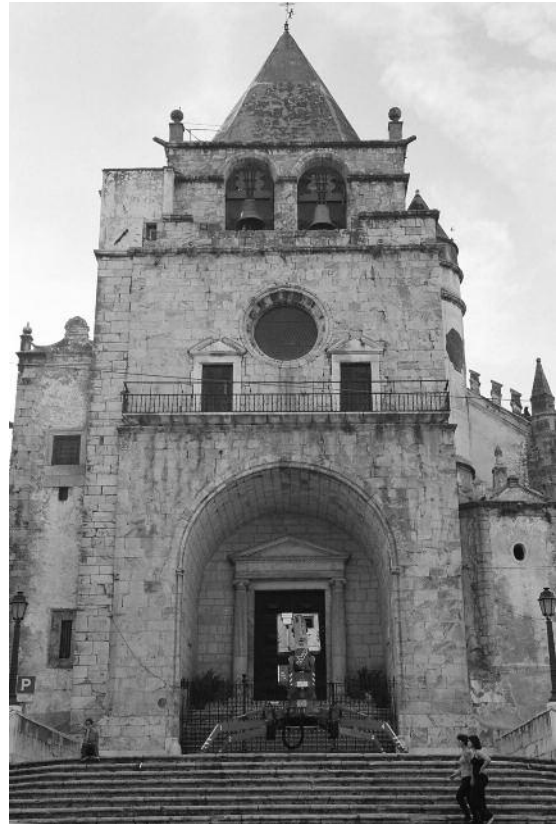
Fig. 1 Church of Nossa Senhora da Assunção before the works of conservation.
