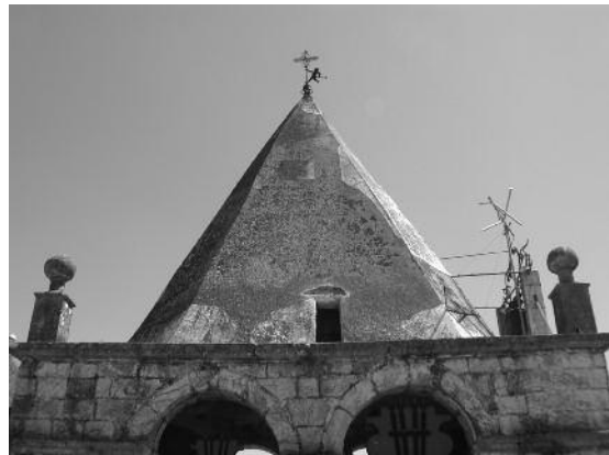
Fig. 3 Initial state of conservation of the pyramidal tower.
