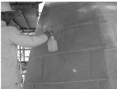
Fig. 18 Detail of the humidifying works.
