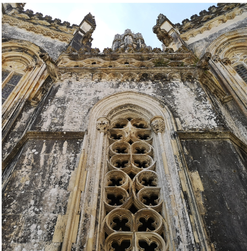
Fig. 1. Batalha Monastery, Portugal. Limestone heavily affected by microbial deterioration and lichenous patinas.
