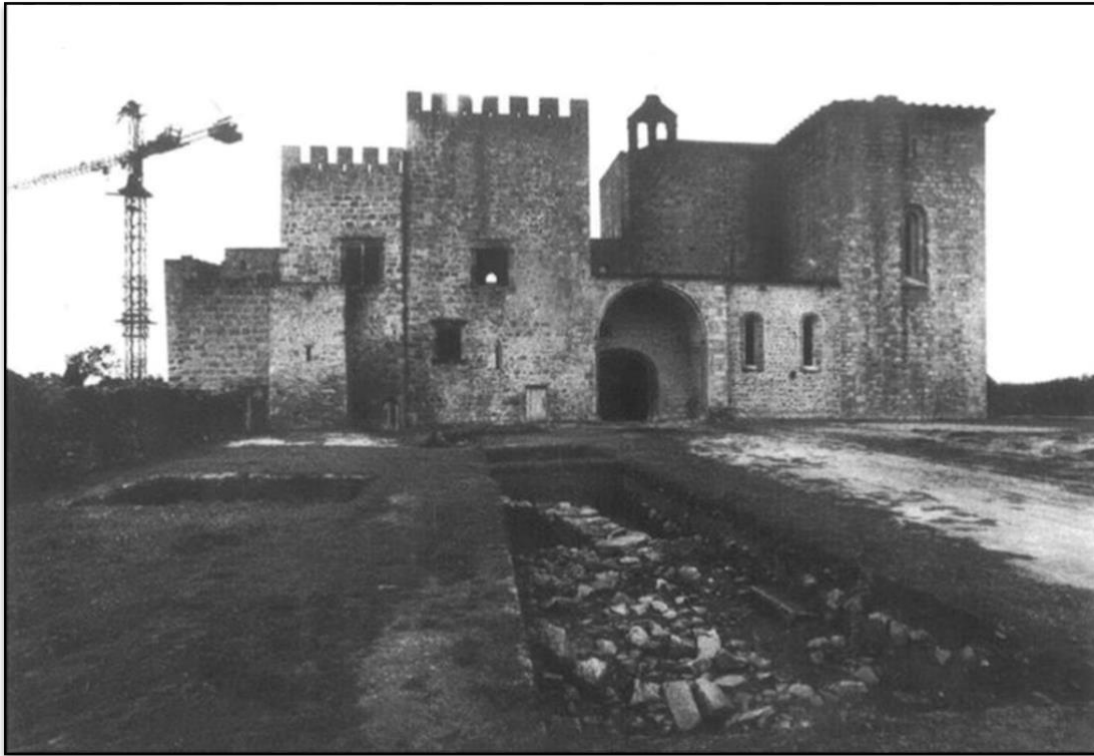
Figure 6 Main façade after excavation (Graça, 1995b, p.67)
