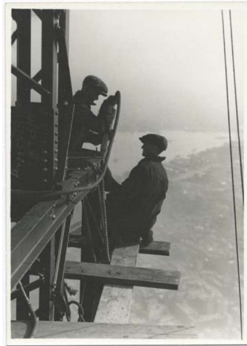
Figure 16 The Miriam and Ira D. Wallach Division of Art, Prints and Photographs: Photography Collection, The New York Public Library. (1931). Two workers riveting a corner beam. Source: https://digitalcollections.nypl.org/items/510d47d9-a90c-a3d9-e040-e00a18064a99 .
