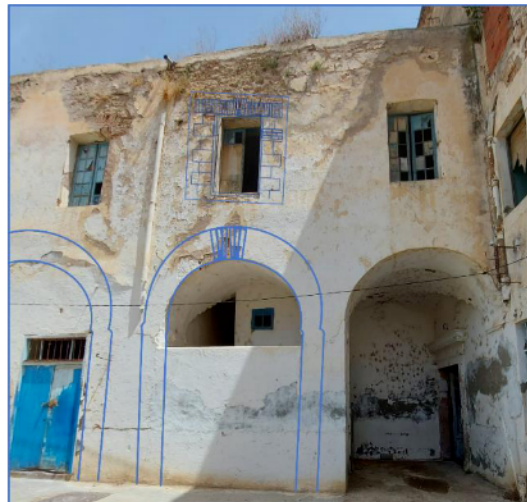
Figure 34: Traçage des arcades. 185
