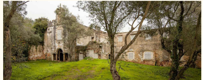
After the intervention
