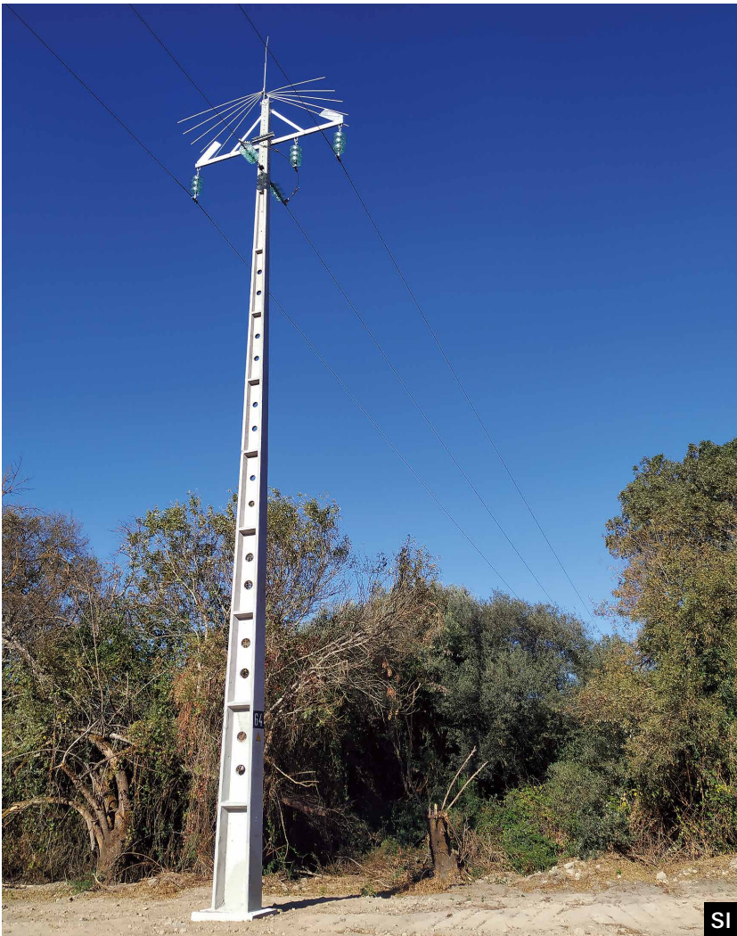
Eco Cross Arms installed in a pole.
