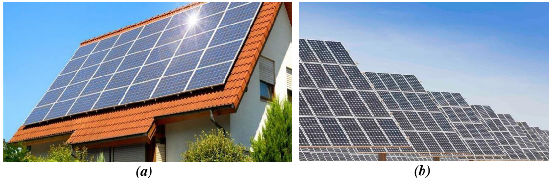
Figure 1.1.4: Photovoltaic panels (a) Photovoltaic panels for electricity generation installed on the roof of a residence. (b) Photovoltaic electricity plant. [4]
