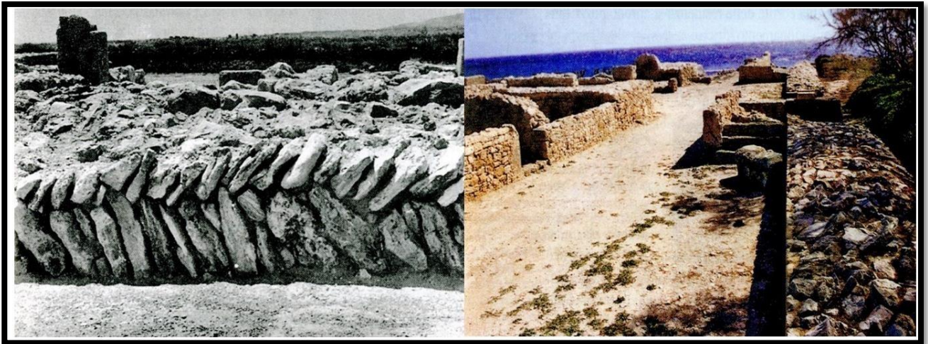
Fig 2.4. On the left: detail of the internal count built with "herringbone" technique. On the right: the south gate and walls with patrol walkway (modified after Bondi 2009).
