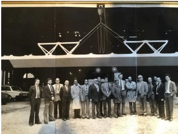
Figure 1 The team who built the deMenil Museum roof (1985): the author (with white hard hat) is next to architect Renzo Piano. The rest of the team are from American contractors, demenil museum and Ove Arup. In the middle is the late Martin Iorns inventor of the laminating process.
