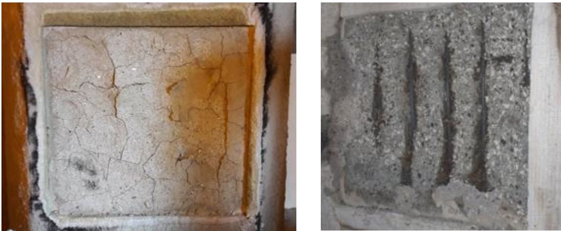
Figure 11 example of 2 real assessment fire tests carried out in 2016 and 2017 in 2 tunnels located along a Paris ring road. These 2 tunnels have been constructed in the years 1970s.
