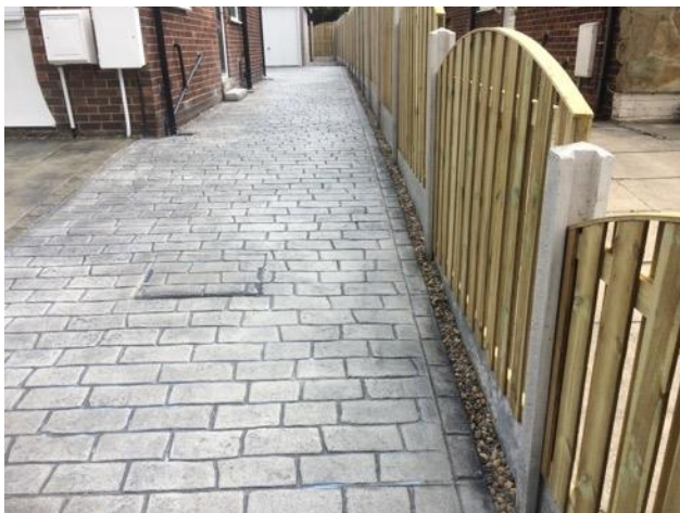
Figure 7 This picture shows an imprinted concrete drive with a 'lead look' finish. This colour can be replicated in a ferrocement long tile to simulate a lead roof of a Church or Cathedral.
