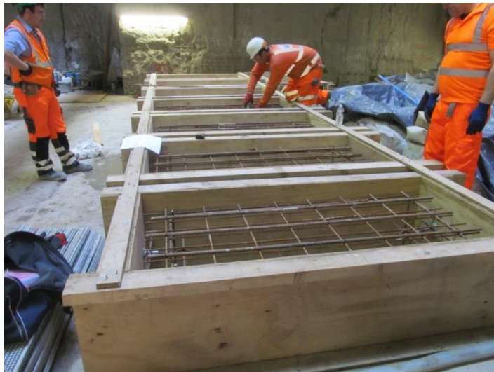
Figure 10 Thermocouple installation on site.
