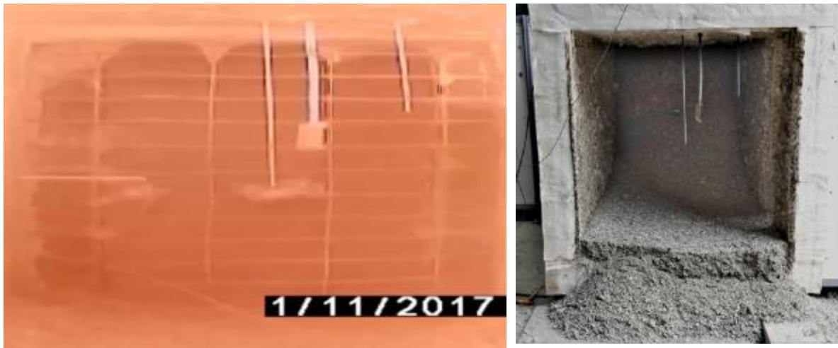
Figure 8 Mobile furnace (slab 5) - Picture from endoscopic camera at the end of the test (52 min) (left). Pile of concrete flakes in the fire chamber after the test (right).
