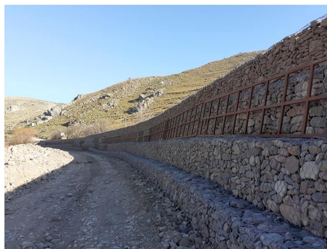
Photo showing the construction "Serazaneti" to stabilize the river bank and to enhance its capacity to accept higher stream power during the flood event (Taken by facebook page "Ο χρούσος")
