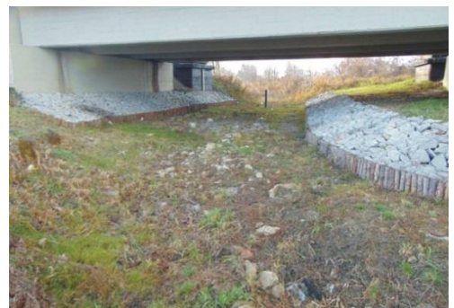
The dry riverbed at the Łysek gauging station (2017).
