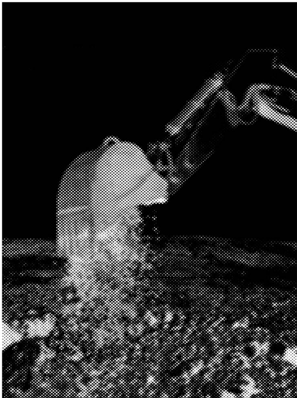
004 Illustration showing hydraulic excavator conducting earthworks. Earthmoving equipment was essential to many Land Artists from the 1960s onwards; Earth became the artist's canvas and earthmoving machines their paintbrushes. © Jared Miguel Fantasia.
