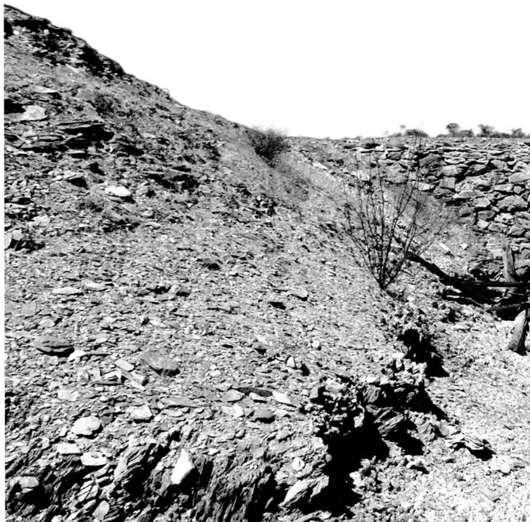
153 Photograph showing one of many infrastructures built for the passage of the railway line from surrounding sedimentary rock available on site. The structure built for the railway integrates with the cliff and also allows the water seepage, coming from above, to pass into the ravine below. © Jared Miguel Fantasia. 2018
