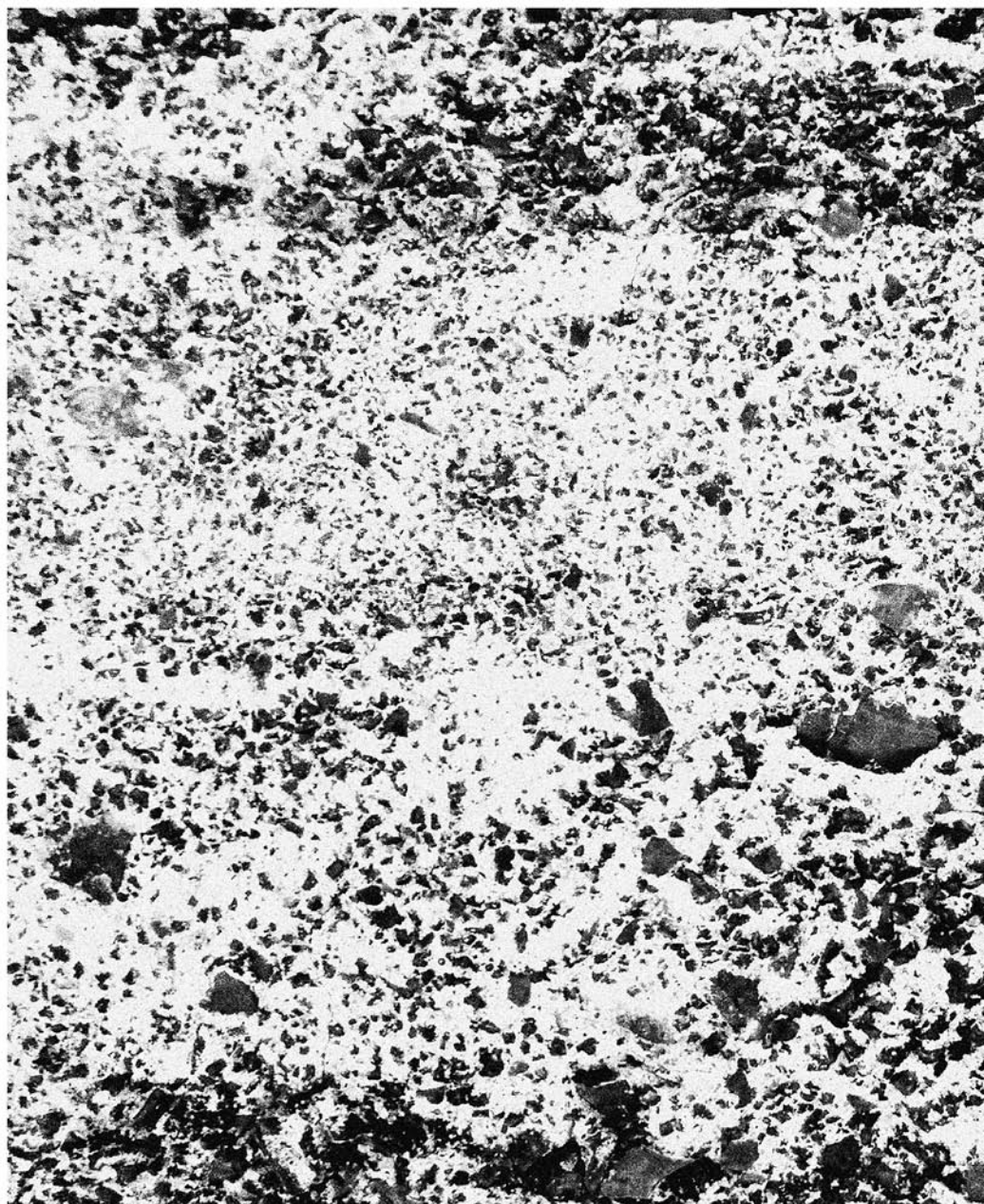
160 Photographic detail (from the previous image 159 on pages 354 to 355) of the concrete structure at the mining tips near the Achada do Gamo ore mills S. Domingos, Portugal. The composition of the structure is much the same as the rest of the concrete structures (built with mining slag) in the surrounding mining area. © Jared Miguel Fantasia. 2018
