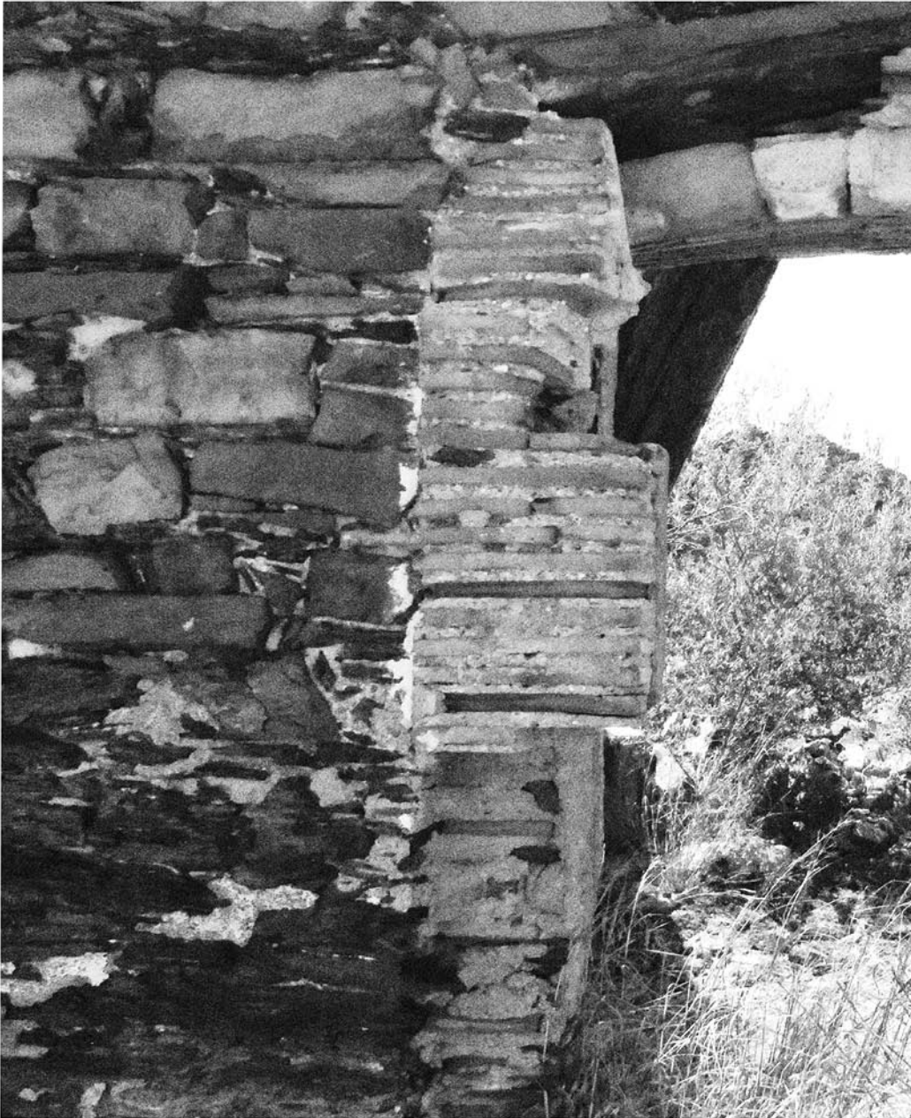
154 Photograph showing a detail of the sedimentary rock that has been used to build most of the surrounding infrastructures in the mining area of S. Domingos. These structures therefore blend into the landscape and, in their decay over time, return to heaps of unorganized matter as they were in the original landscape prior to their use. © Jared Miguel Fantasia. 2018
