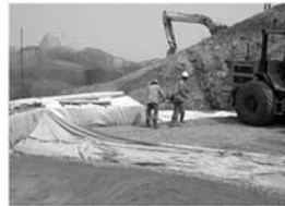
Compacting granular drainage blanket wrapped in Polyfelt® TS50 geotextile filter
