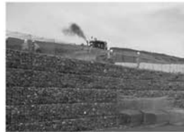
Construction of gabion facing
