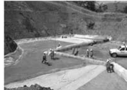
Placing Polyfelt® PEC geocomposite reinforcement across reinforced soil wall
