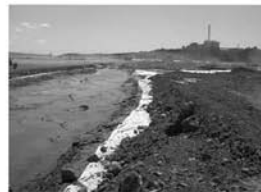
Partial closure of the mine tailings pond
