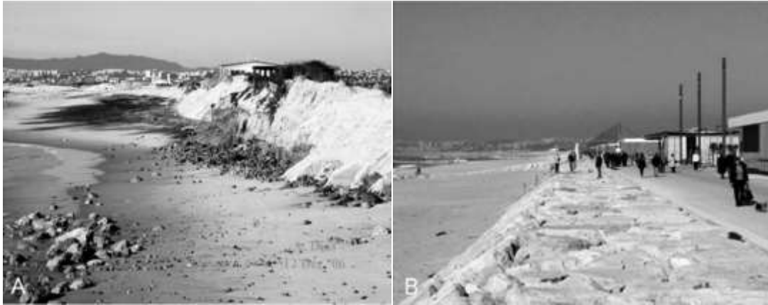
Figure 17: Views of the Costa da Caparica beach deprived of sand in 2006 (A; courtesy of Alveirinho Dias) and the beach and its marginal strip after the last major intervention in 2014 (B). This arrangement has remained substantially constant since 2010, with only some interventions in the support structures and the replacement of small amounts of sand that are lost annually (a few hundred thousand cubic metres per year from approximately 2 km of beach).
