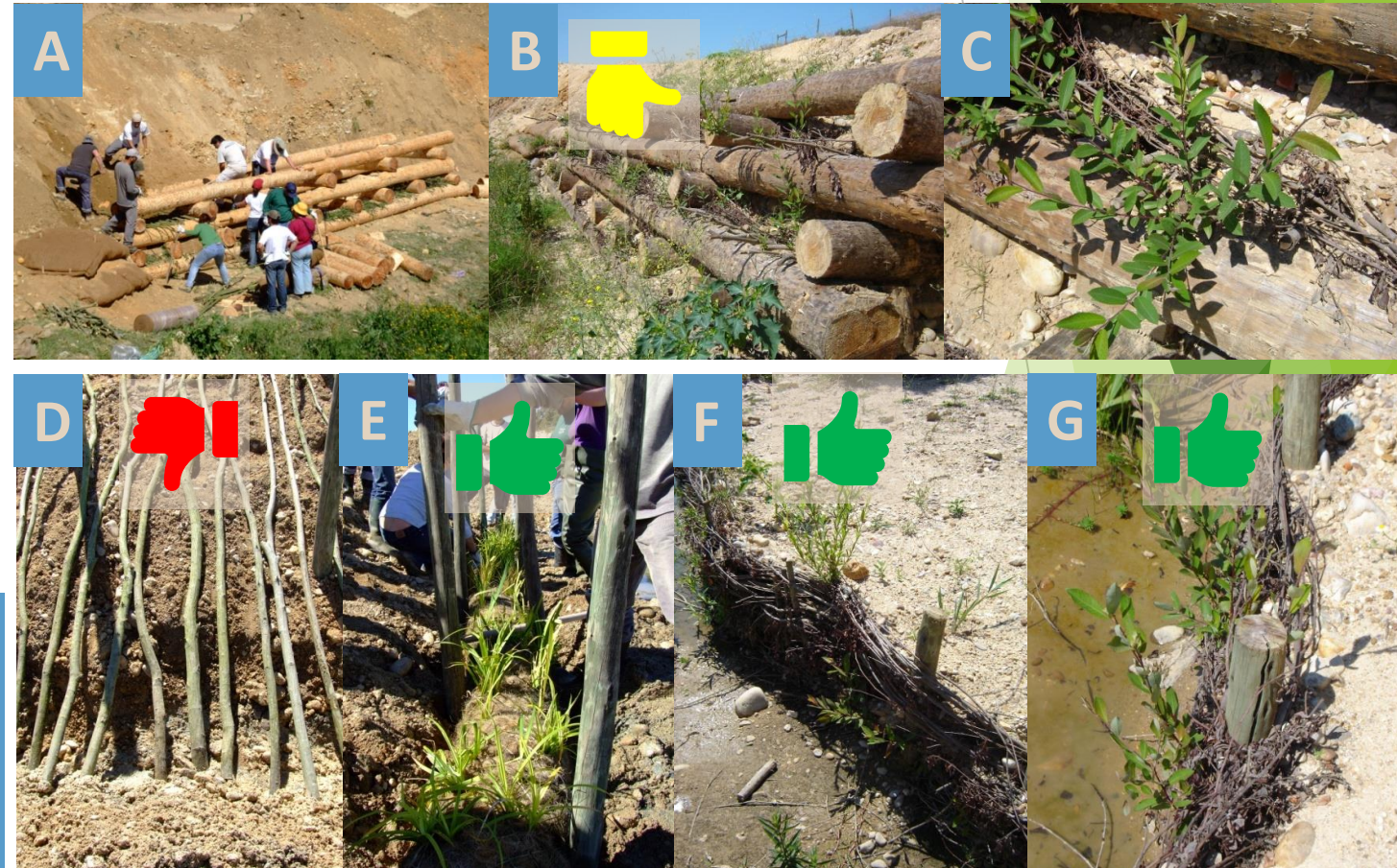
A, B e C: Cribwall D: Brush mattress E: planted coconut fiber rolls F: Wattle fences G: Live fascines
