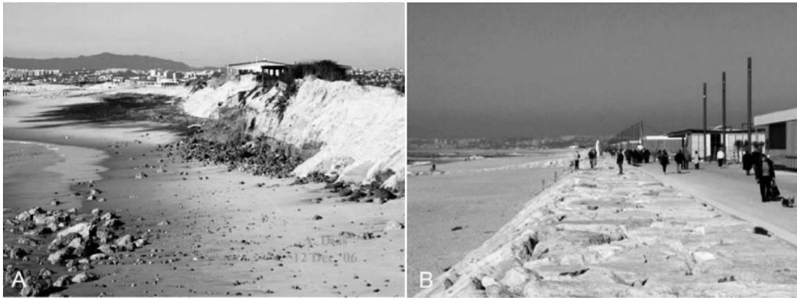
Figure 15: Views of the Costa da Caparica beach deprived of sand in 2006 (A; courtesy of Alveirinho Dias) and the beach and its marginal strip after the last major intervention in 2014 (B). This arrangement has remained substantially constant since 2010, with only some interventions in the support structures and the replacement of small amounts of sand that are lost annually (a few hundred thousand cubic metres per year from approximately 2 km of beach).
