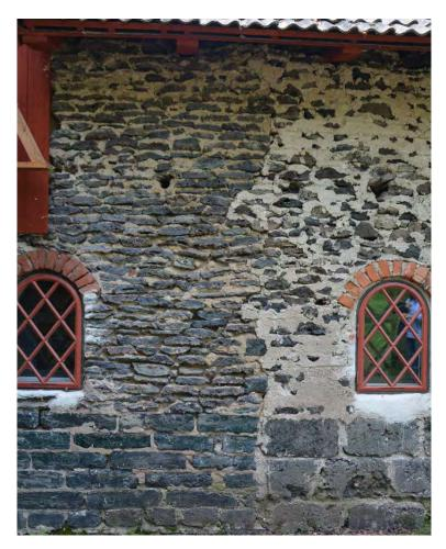
Figure 4. At the Unesco site of Engelsberg can buildings with different types of cast masonry slag blocks be studied.
