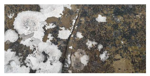
Figure 2. Ethyl silicate mortar repairs carried out to a broken stone in 1996. This image, taken 23 years later in 2019, shows the stone still wet after rain. The mortar repair, now detaching due to movements in the joined stone, achieves both requirements of having good wet colour and a balanced recolonization of biota, in this case two forms of crustose lichen.
