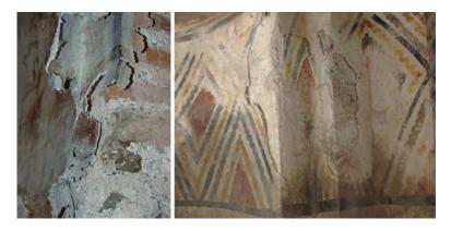
Figure 1. Detachments and loosening of the mortar layers from murals' substrate
