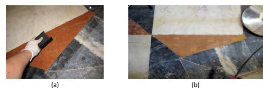
Figure 2. Finishing of the surface: (a) polishing using different wet sandpapers; (b) application of fluid pastes to fill the pores that still prevail
