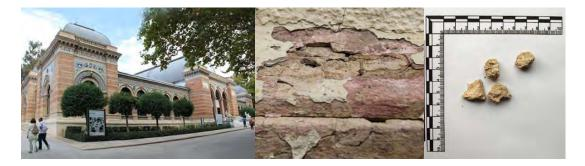
Figure 5. Main facade of the Velazquez Palace. Detail of the run profile decoraration where the sample was taken.
