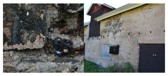
Figure 2 left. Slag stone with a glassy structure. Figure 2 right. A barn made of slag chips.
