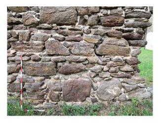
Figure 2. Part of the test wall with rubble stone of different size and shape and joints in parts deeply eroded
