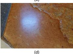
Figure 11. Evaluation of the intervention after one year: (a) stone slab just after restoration; (b) the same slab after a year of use; (c) stone partly restored, where the dirtiness on the unrestored holes is visible; (d) surfaces of the stone and of the reintegrated parts in stucco with some visible scratches
