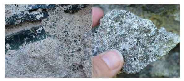
Figure 3 left. Cast slag bocks and slag mortar where the slag particles are rather big. Figure 3 right. A slag mortar with both sand and slag granulates.
