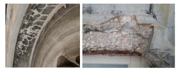
Figure 6. Detailed view of the façades. a) Shrinkage cracks of the natural cement mortars, b) Spall revealing a highly corroded rebar.
