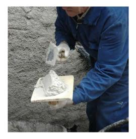
Figure 2: Rendering with warm mortar (2009)
