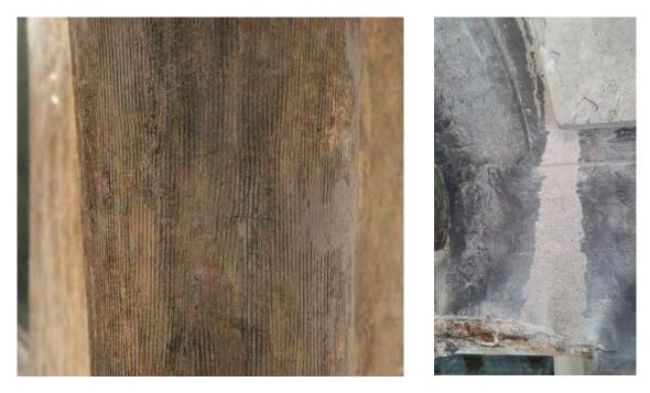
Figure 4. Detailed view of the façades. a) Chiselled finishing, b) Black crust under the paint.
