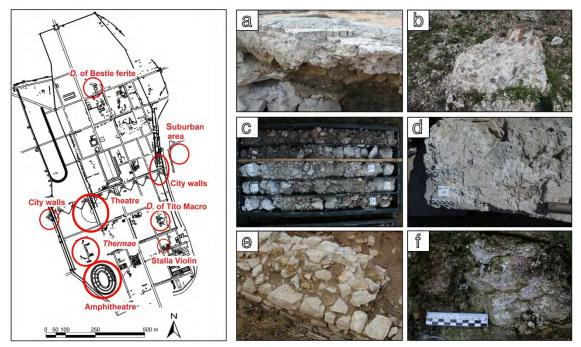
Figure 1. Aquileia. Plan of the investigated archaeological sites. a) mosaic bedding screed at *Domus* of Bestie ferite; b) collapsed vault of *Thermae Felices Constantinianae*; c) core drilling in theatre foundation platform; d) jointing mortars of the amphiteatre; e) wall of eastern fluvial bank; f) joint mortar with shell aggregates of Bizantine city walls.
