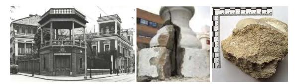
Figure 14.: Exterior view of the Cerralbo Palace. Garden pavilion. Detail of the damage of the balustrades of artifical stone.
