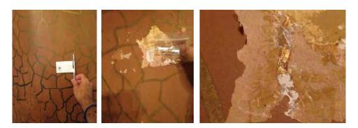
Figure 22a. Current paint. Figure 22b. Extraction of micro-samples. Figure 22c. Detail of the golden leaf appeared in the selective stripping.
