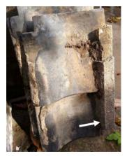
Figure 1a. The old Japanese roof-tiles with cement
