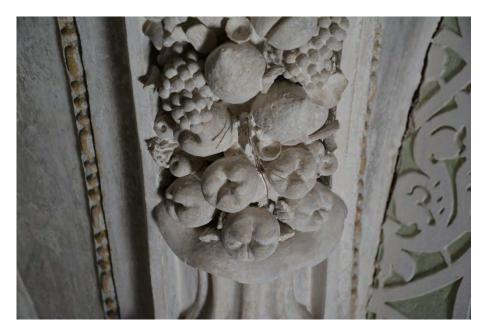
Figure 2. Bottom part of a rib formed by two L shape mortar profiles enclosing the vase with the fruit. Transfers from the rib to the plain vaulted surfaces are decorated by a bead moulding.
