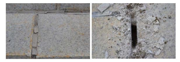
Figure 2. Foley Courthouse, Albany, New York, built 1932 to 1934. Some pavement mortar failures manifested themselves as a thin layer of dry, hardened mortar above a layer of wet, disaggregated mortar, presumably corresponding with the depth within the joint at which mortar was frozen while saturated. Photos by Chad Lausberg
