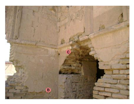
Figure 4: sample locations of the plasters B and C in the western corner of room 6
