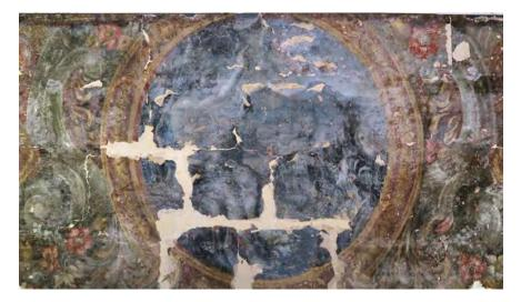
Figure 1. Detail of Baroque painting on east wall of the Chapel at Palazzo de la Salle. Note the characteristic pattern of painted plaster detachment and loss along the joins between ashlar support (Department of Conservation and Built Heritage, University of Malta, 2018).
