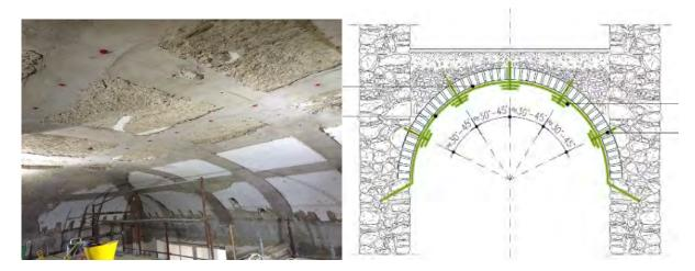
Figure 9. Intrados strengthening of vaults
