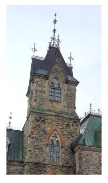
Figure 1. East Block Parliament Hill, Ottawa, Ontario, built 1859-1866, the sloped elements (below the windows) of the northwest tower four years after repointing of the freeze-thaw damaged areas with polymer modified repointing mortar, 2017. Photo by Michael Edison.
