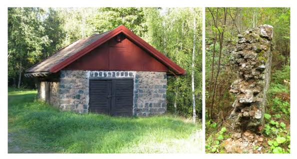
Figure 1 left. BF slag mortars and masonry blocks of cast slag in forge shop at Flatenbergs hyttan. The repair above the door is made with pure lime mortar. Other parts of the building still have the original mortar. Figure 1 right. Example from Schisshyttan the ruin of a steel workshop constructed in 1763.
