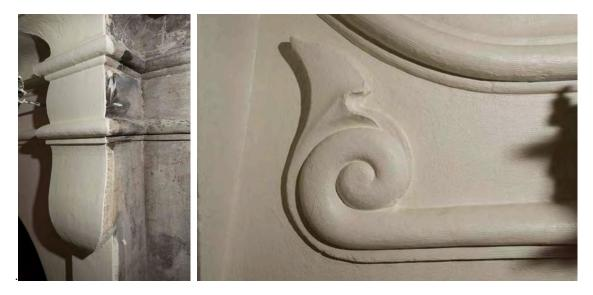
Figure 16. The water-based polyurethane coating dedicated to preserving the concrete unfortunately did mask the incredibly detailed surface of the façade. Picture by Dominique Bouchardon.
