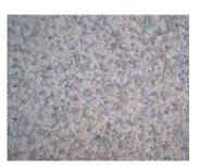
Figure 1 – Façade of LNEC main building covered with *marmorite* render: a) General view; b) Detail of *marmorite*
