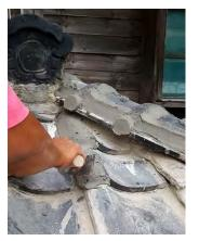
Figure 1b. Plastering the lime mortar on old Japanese rooftiles
