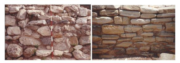
Figure 1. Clay mortar between rubble walls in Khirokitia and Kalavasos-Ayios Dhimitrios
