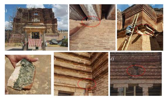
Figure 1: (a) - Front view of the entrance tower, (b) to (e) - sampling locations inside the tower, (f) - a detached sample from the top of the tower
