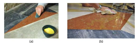
Figure 10. Protection of the external surface: (a) application of a mixture of waxes; (b) final polishing of the surface
