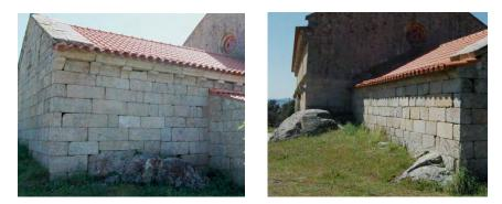
Figure 7. Granite blocks unexcavated, part of the walls: (A) Approximately with three meters on the North façade of the main chapel. (B) One small and the other with a length of approximately three meters on the South facades of the main chapel and nave.
