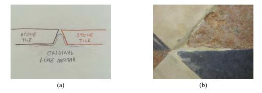
Figure 4. Restoration of the joints: (a) section of the shape of the slabs on the edges; (b) detail of one of the fillings with lime mortar
