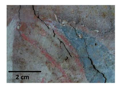
Figure 2: Detail of detached painted plaster in the wall painting at Palazzo de la Salle. The detachment between plaster and wall is ~1-2 mm wide (Department of Conservation and Built Heritage, University of Malta, 2016).
