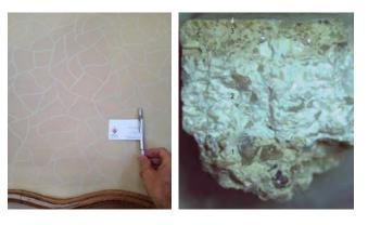
Figures 13a and 13b. Wall presently painted, and coloured lime stucco section.
