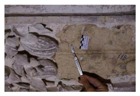
Figure 3. Top part of a rib with some fruit pieces fallen out showing the first coat and the remains of the adhesive mortar II layer on sides and between the fruits. The scalpel points at the position of sample MCL1.
