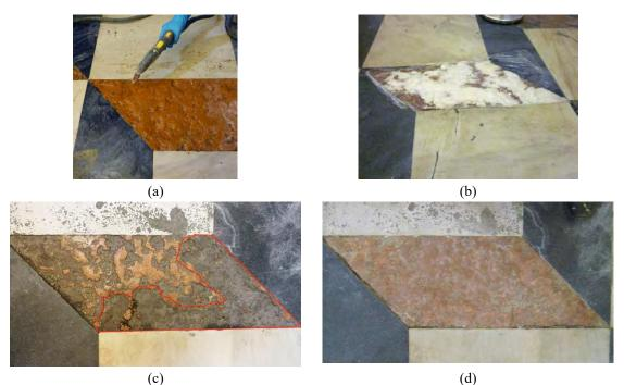
Figure 3. Cleaning of the paving stones: (a) using the steam cleaner; (b) application of paper pulp with ammonium bicarbonate; (c) stone slab before cleaning; (d) the same slab after cleaning
