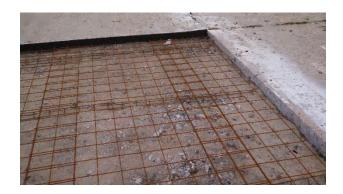
Figure 6. Typical prepared repair area, with welded wire mesh placed for reinforcement. Photo by the author.
