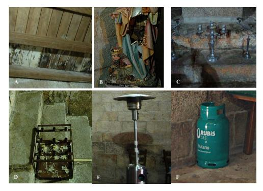
Figure 9. (A) Actual state of the ceiling in the sacristy with water infiltrations. (B) Wooden polychromed sculpture hollowed by insects infestation. (C) and (D) Candlesticks placed on the stairs of the main chapel and when litten, the hot wax pours onto the granite floor. (E) Gas heater. (F) Butane gas cylinder
