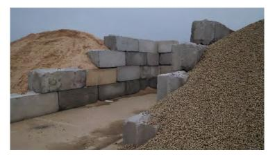
Figure 4. Onsite storage of fine and coarse aggregates. Photo by the author.
