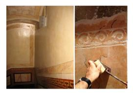
Figure 19. Hot-ironed stucco's technique, applying a hot iron tool over the surface of the lime mortar, that ends up by giving a shiny and smooth result, as shown in the pictures.
