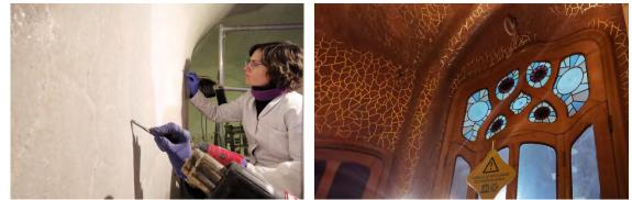
Figure 28. Restoration works, stripping the paints and recovering the original coloured lime stuccoes and their sgraffitos. Figure 29. Fireplace Room already restored, with the original finishes recovered.
