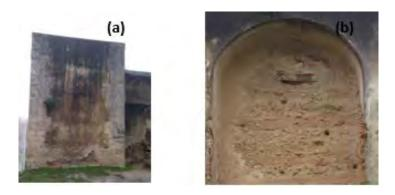
Figure 5 – Gil Vicente's School: (a) small tower with stone masonry corners and rammed earth and (b) rammed earth section of the Wall
