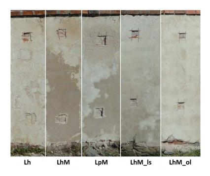
Figure 2. Experimental renders 12 months after application (LhM\_ls and LhM\_ol) and 24 months after application (Lh, LhM and LpM).
