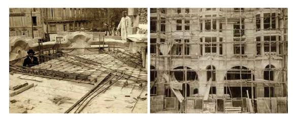
Figure 1. Pictures by Clément Maurice [11] [12]. a) The newly patented Hennebique reinforced concrete was employed. b) Overview of the worksite.
