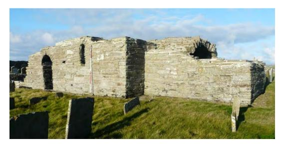
Figure 1a (above) – Crosskirk Tuquoy from the south-east. Note the putlog socket between nave doorway and window. Scale 500mm; photograph Mark Thacker.
