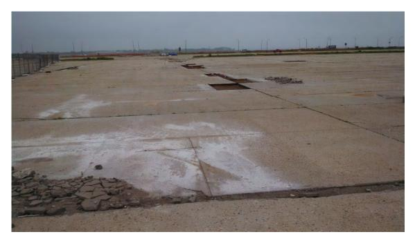
Figure 3. Typical damaged pavement areas, resulting from placement and removal of Hurricane Sandy debris. Photo by the author, 2014.
