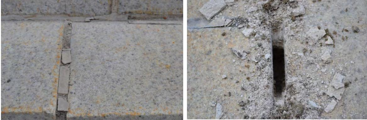
Figure 2. Foley Courthouse, Albany, New York, built 1932 to 1934. Some pavement mortar failures manifested themselves as a thin layer of dry, hardened mortar above a layer of wet, disaggregated mortar, presumably corresponding with the depth within the joint at which mortar was frozen while saturated. Photos by Chad Lausberg
