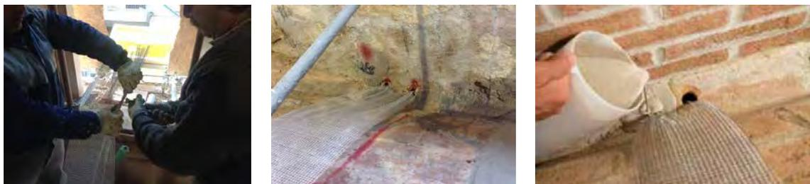
Figure 5. Double side spikes for anchoring
