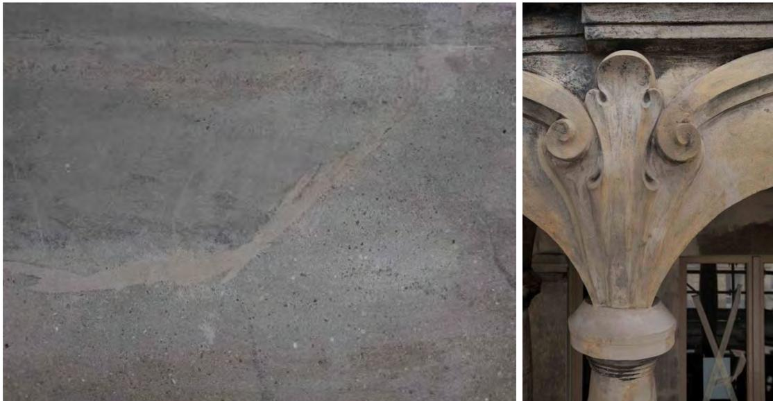
Figure 15. Cracks and spalls were repaired using slurries and natural cement-based mortars. Picture by Dominique Bouchardon
