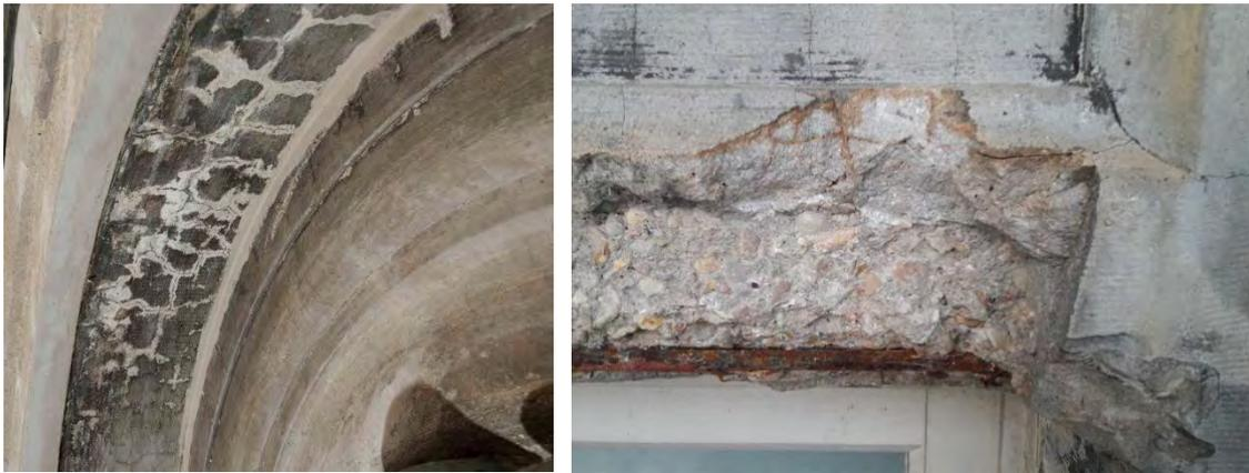
Figure 6. Detailed view of the façades. a) Shrinkage cracks of the natural cement mortars, b) Spall revealing a highly corroded rebar.
