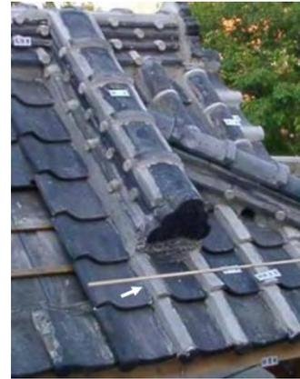
Figure 1c. The old Japanese roof-tiles with lime mortar [22]
