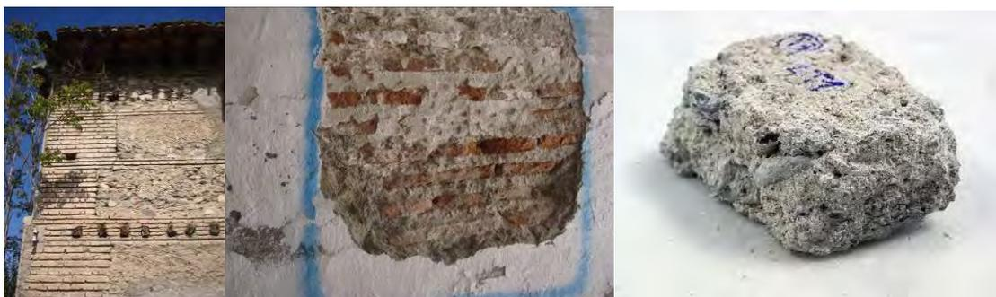
Figure 4. Mixed masonry walls
