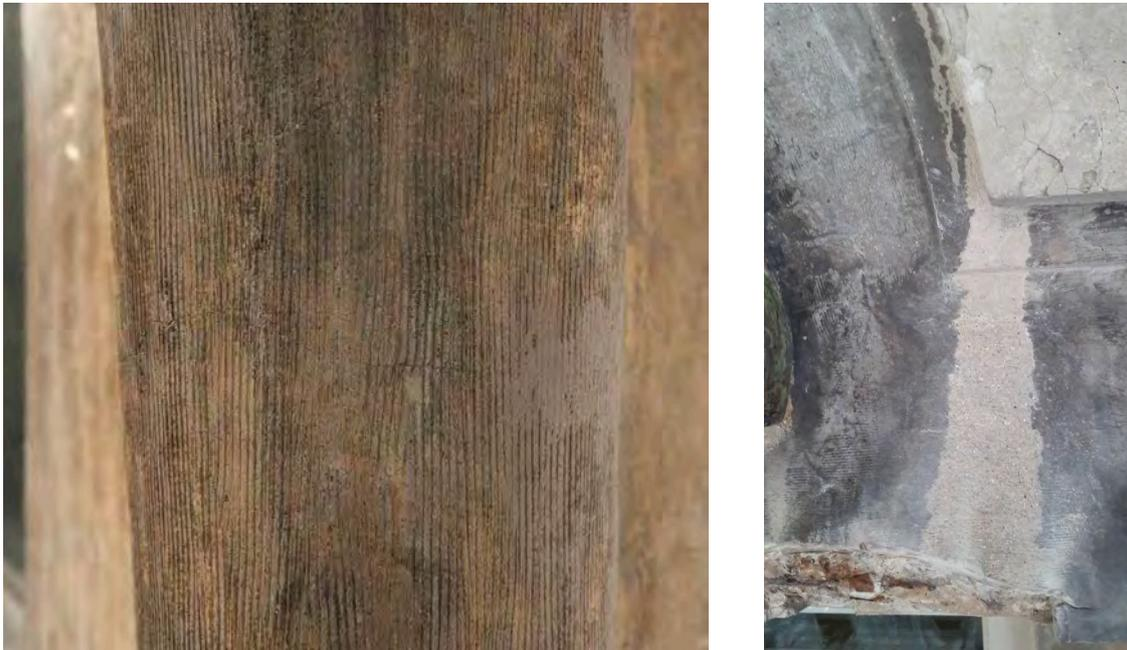
Figure 4. Detailed view of the façades. a) Chiselled finishing, b) Black crust under the paint.
