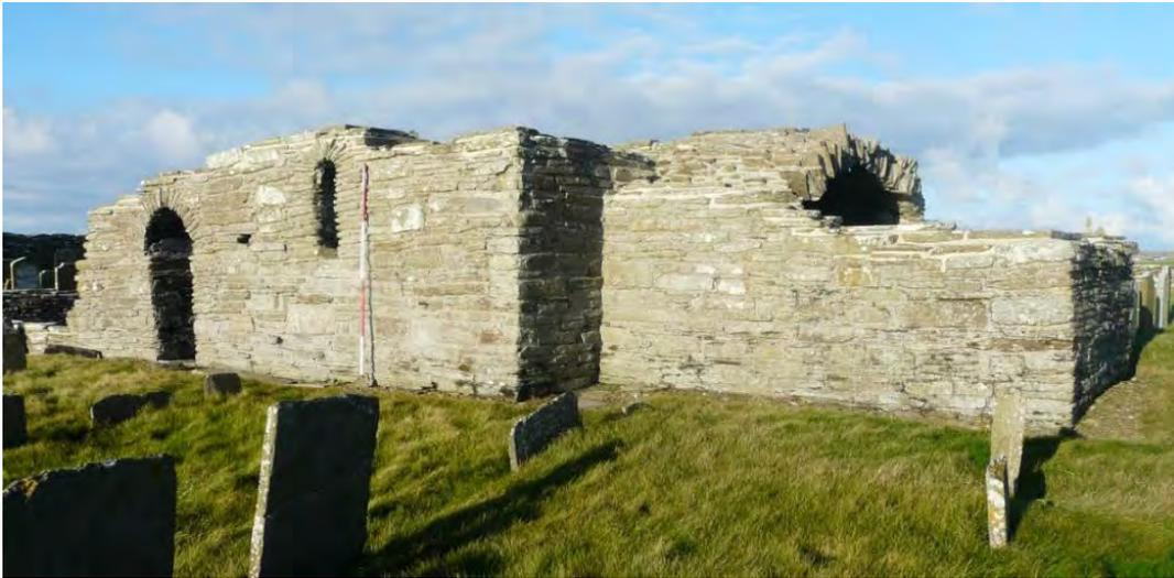
Figure 1a (above) – Crosskirk Tuquoy from the south-east. Note the putlog socket between nave doorway and window. Scale 500mm; photograph Mark Thacker.
