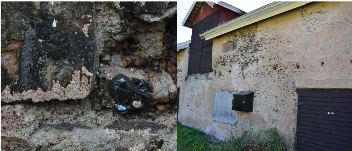
Figure 2 left. Slag stone with a glassy structure. Figure 2 right. A barn made of slag chips.
