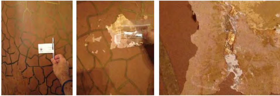
Figure 22a. Current paint. Figure 22b. Extraction of micro-samples. Figure 22c. Detail of the golden leaf appeared in the selective stripping.
