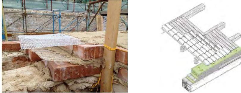
Figure 8. Ring beams reinforced with interposition in bed-joints of galvanized steel fiber strips
