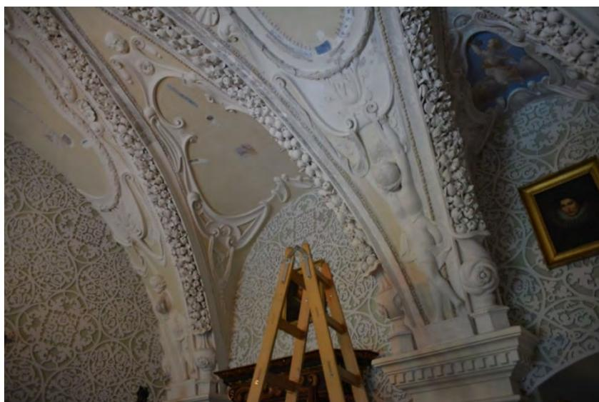
Figure 1. Stucco decorated vaulted ceiling of the Great Chamber at Červená Lhota castle at the stage of detailed surveying – a preparatory phase for uncovering the frescos and cleaning the coatings.
