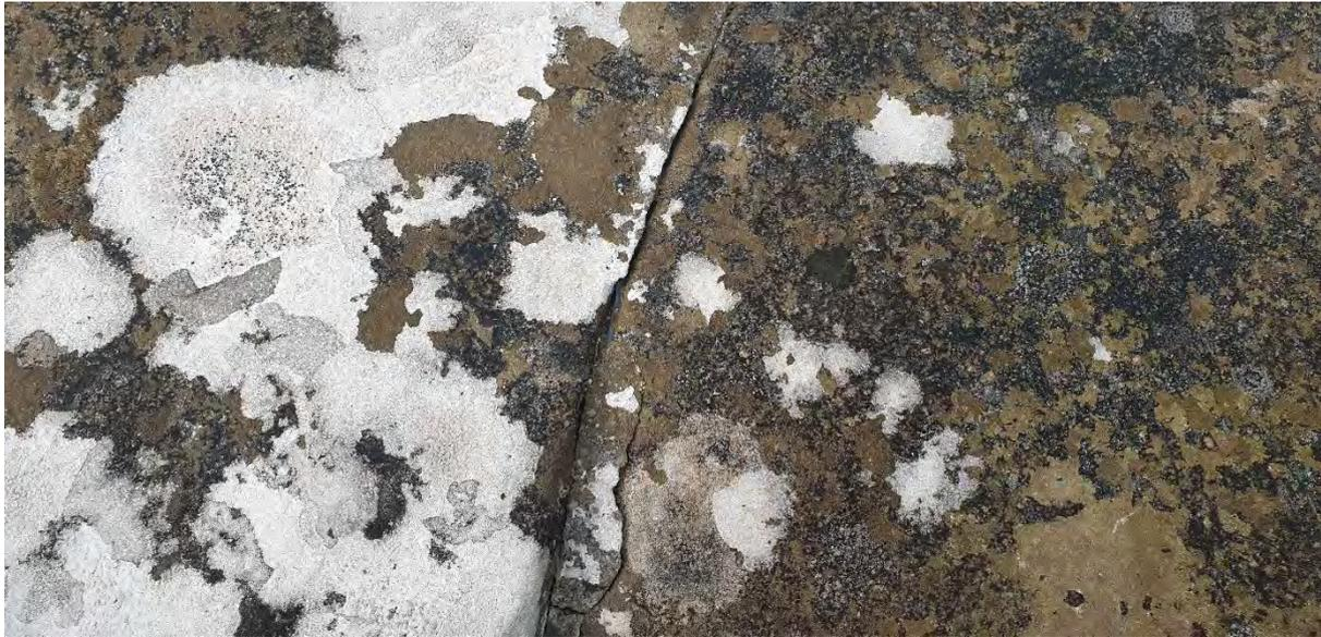
Figure 2. Ethyl silicate mortar repairs carried out to a broken stone in 1996. This image, taken 23 years later in 2019, shows the stone still wet after rain. The mortar repair, now detaching due to movements in the joined stone, achieves both requirements of having good wet colour and a balanced recolonization of biota, in this case two forms of crustose lichen.
