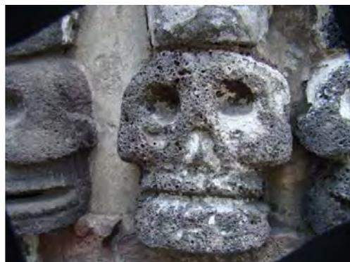
Figure 3. Detail of the Aztec altar of skulls, where original plaster is lost and stone presents decay because of the presence of soluble salts from the lime/cement joints. STROM/INAH 2009.
