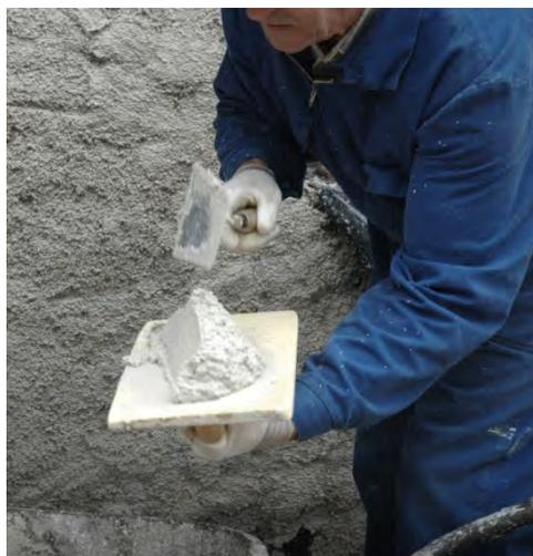
Figure 2: Rendering with warm mortar (2009)
