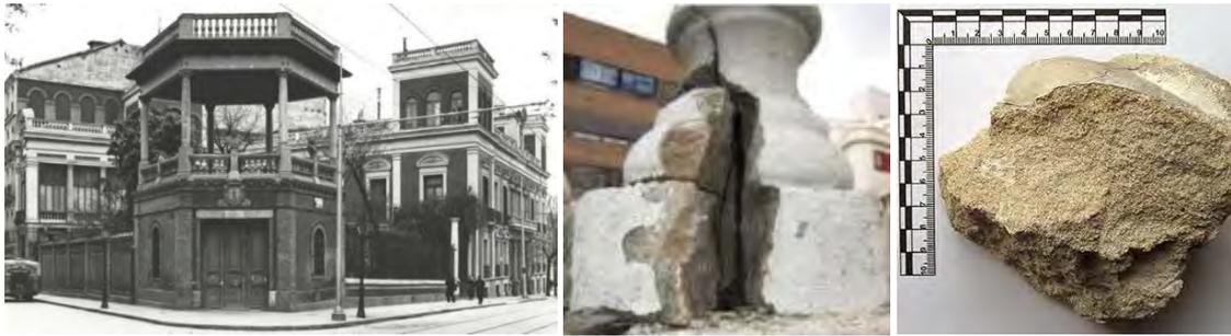
Figure 14.: Exterior view of the Cerralbo Palace. Garden pavilion. Detail of the damage of the balustrades of artificial stone.
