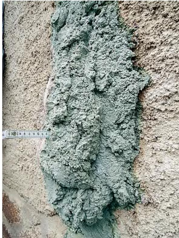
Figure 3. Hot applied mortar (HAM) in mixture H3, with pumice, allows a thick package of mortar applied in one step because of very fast setting
