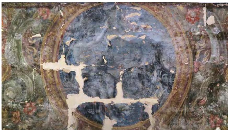
Figure 1. Detail of Baroque painting on east wall of the Chapel at Palazzo de la Salle. Note the characteristic pattern of painted plaster detachment and loss along the joints between ashlar support (Department of Conservation and Built Heritage, University of Malta, 2018).
