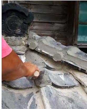
Figure 1b. Plastering the lime mortar on old Japanese roof-tiles
