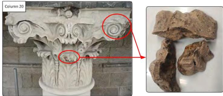
Figure 2. Portland stone at The Four Courts showing old mortar repairs made with crushed Portland stone - Figure 3.
