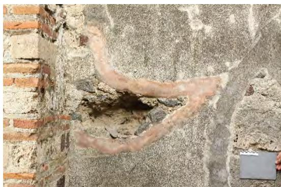
Figure 1. Reddish repair mortar No. 2002 in the Casa del Labirinto. (Fraunhofer IBP, 2017)
