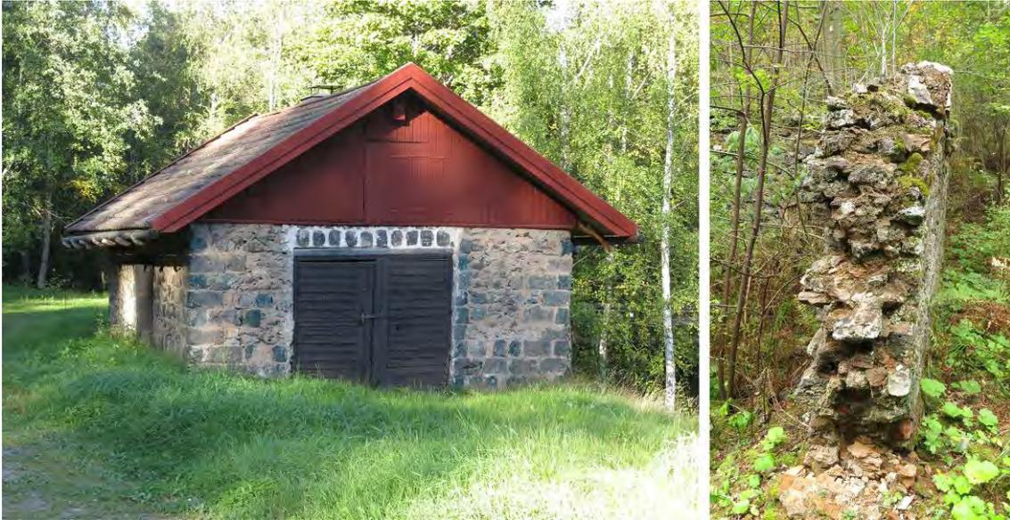
Figure 1 left. BF slag mortars and masonry blocks of cast slag in forge shop at Flatenbergs hyttan. The repair above the door is made with pure lime mortar. Other parts of the building still have the original mortar. Figure 1 right. Example from Schisshyttan the ruin of a steel workshop constructed in 1763.
