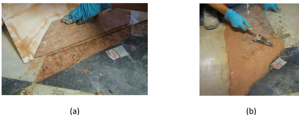
Figure 7. Application of the final layer: (a) fitting the previously moulded stucco marble paste; (b) compacting the surface with a trowel.
