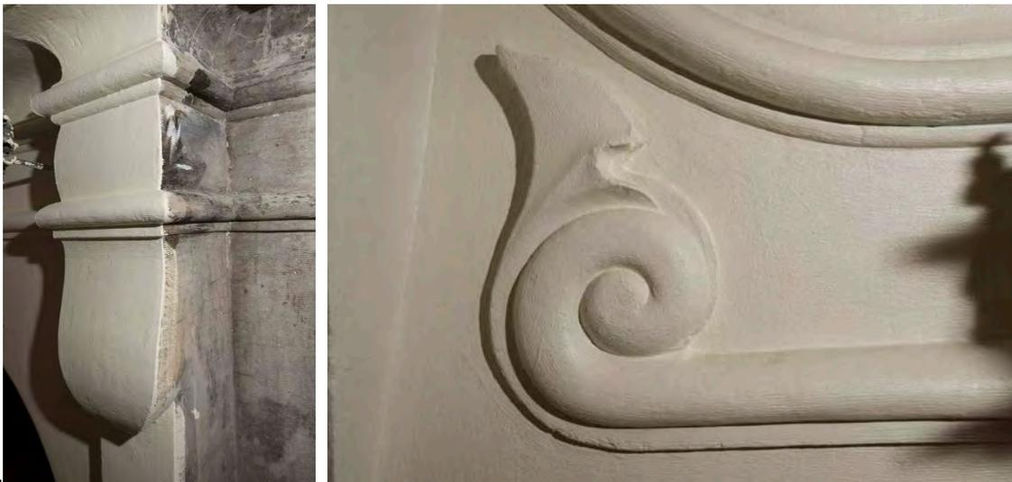
Figure 16. The water-based polyurethane coating dedicated to preserving the concrete unfortunately did mask the incredibly detailed surface of the façade. Picture by Dominique Bouchardon.
