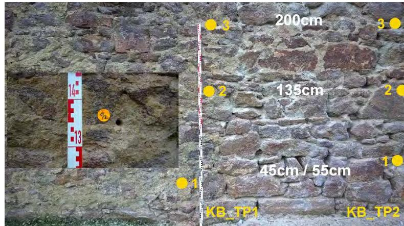
Figure 6. Test area at the historic wall with sampling points for salt and moisture investigations
