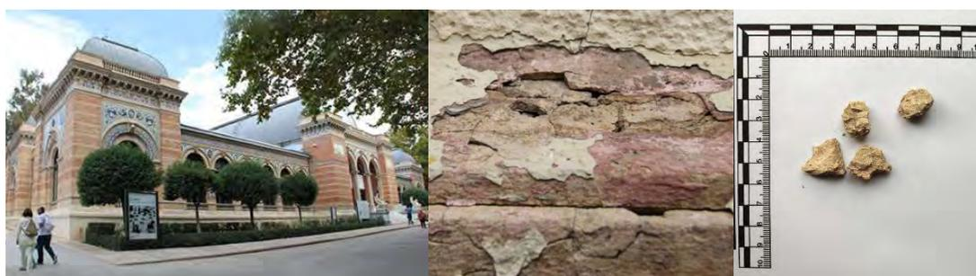
Figure 5. Main facade of the Velazquez Palace. Detail of the run profile decoration where the sample was taken.
