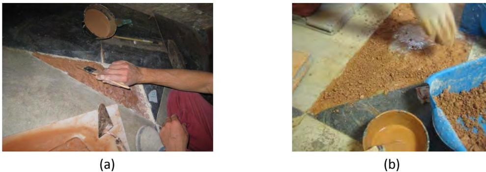
Figure 6. Application of the preparation layers: (a) stucco grout; (b) stucco mixed with gravel.
