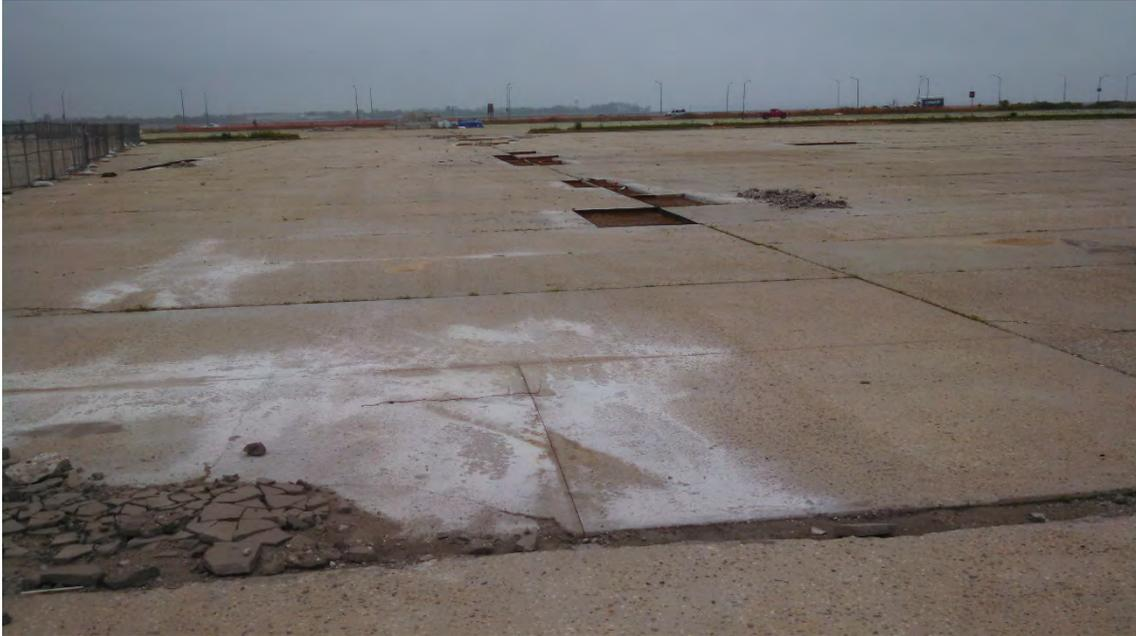
Figure 3. Typical damaged pavement areas, resulting from placement and removal of Hurricane Sandy debris.
