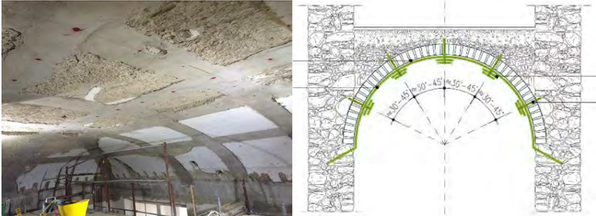
Figure 9. Intrados strengthening of vaults
