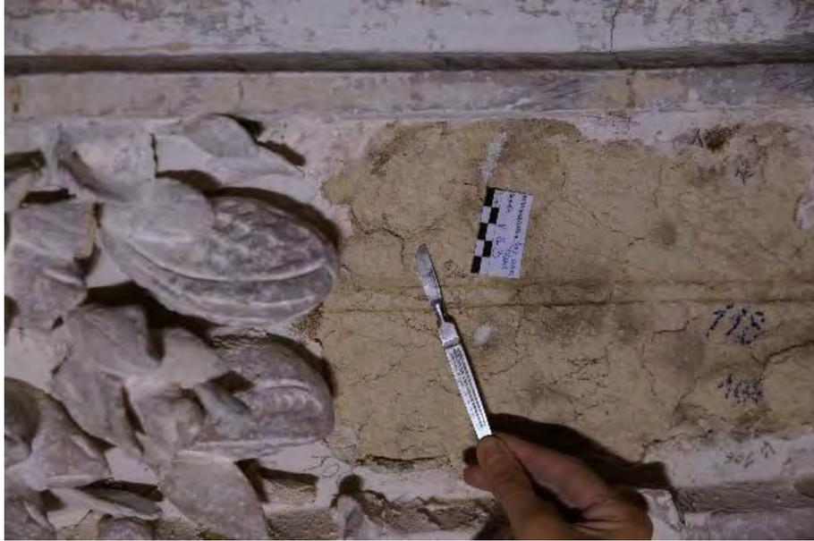
Figure 3. Top part of a rib with some fruit pieces fallen out showing the first coat and the remains of the adhesive mortar II layer on sides and between the fruits. The scalpel points at the position of sample MCL1.
