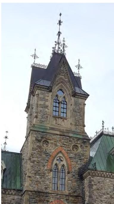
Figure 1. East Block Parliament Hill, Ottawa, Ontario, built 1859-1866, the sloped elements (below the windows) of the northwest tower four years after repointing of the freeze-thaw damaged areas with polymer modified repointing mortar, 2017. Photo by Michael Edison.
