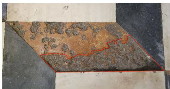
Figure 2. Detail of one damaged paving stone: the red line shows the part to be restored with stucco marble
