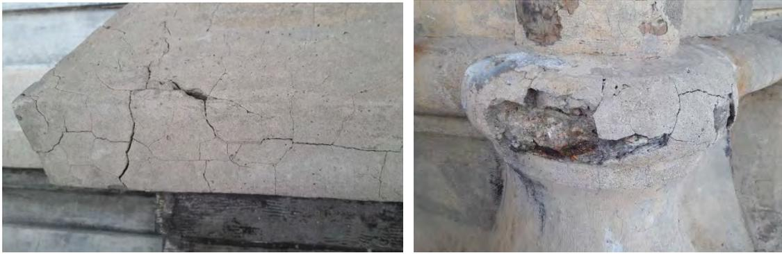
Figure 5. Detailed view of the façades. a) Shrinkage cracks of the natural cement mortars, b) Spall revealing a highly corroded rebar.
