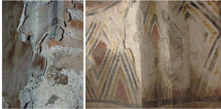
Figure 1. Detachments and loosening of the mortar layers from murals' substrate
