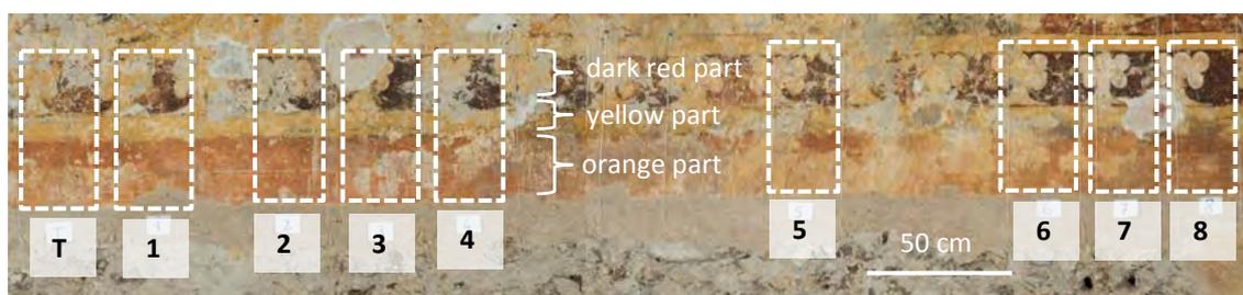
Figure 2. The nine test areas on the east wall with orange, yellow and dark red parts
