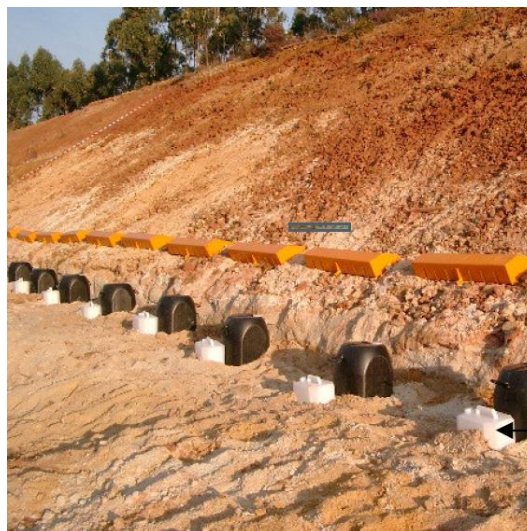
Figure 3 Example of installation of collecting boxes (from de Assunção Alho, 2006)
