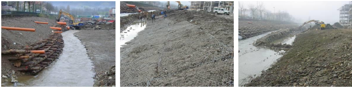
Double crib wall, gabion mattress and bush mattress (source: P. Sangalli )
