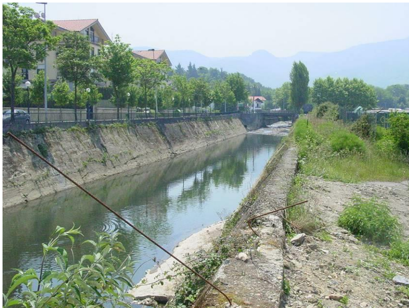
Pre-operational situation. The channel is formed by a trapezoidal cross section made of concrete
