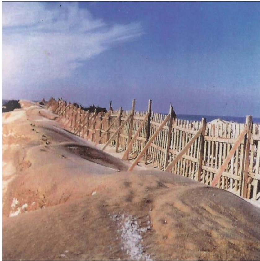
The wooden fences constructed to stabilize sand dune movement in 1961 (Archive of General Directorate of Forestry, 2012)
