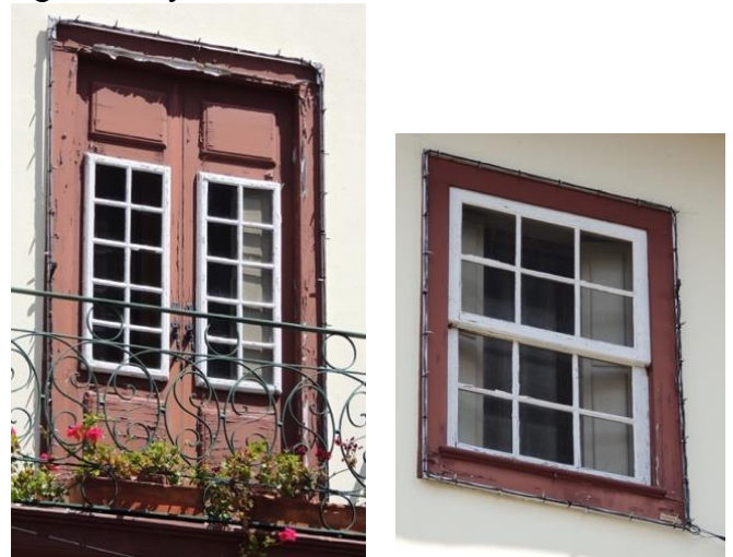
Figure 3: Caption of frames of south façade of Pousada Nossa Senhora das Oliveiras. New double glazing windows and doors painted with two different colours. Luísa Ghignatti, 2015.
