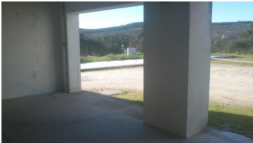
Figure 6: Selected site to install the VRFB Microgrid (Polo da Mitra)
