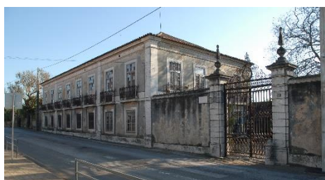
Figure 5. Quinta Alegre: preservation of the manor house and extension to house an intergenerational residential unit.
