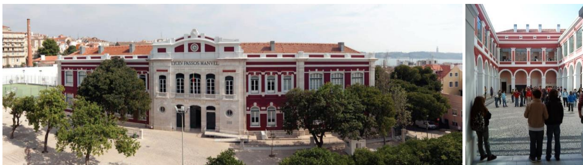
Figures 3 and 4. Passos Manuel Lyceum, after intervention: main façade and recreational use by students in the historic environment of the restored enclosed courtyard.
