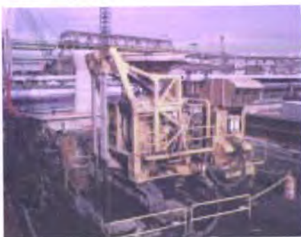
Above: Hydrocutter operating on the Boston Central Artery Project along active rail tracks at North Station.
