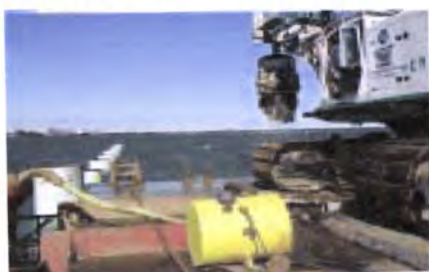
A bridge being constructed over Cedar Creek. A highly protected Salmon spawning tributary to the Columbia River.
