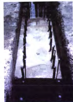
Top: A typical bentonite diaphragm wall covered with contaminated Bentonite / Concrete.
