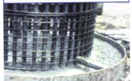
Below: A 12 ft. diameter pile dug in water sensitive clay with the Vinyl System.
