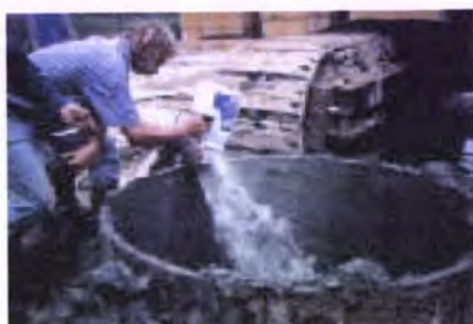
Above: SlurryPro CDP being added directly to a bored pile in Bangkok.
