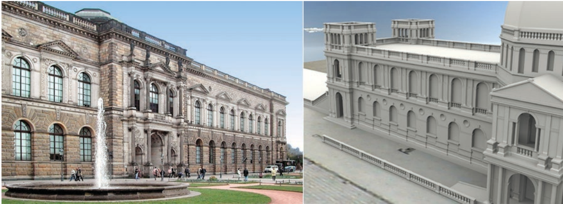
Fig. 33 Reconstruction of the ground storey of Gottfried Semper's design for a picture gallery in front of the residential castle (time-cut no. 13; cf. fig. 31) by borrowing motifs (medallions, cornices, pillar arcades) from the outer façade of the executed building (virtual model 2009-11).
