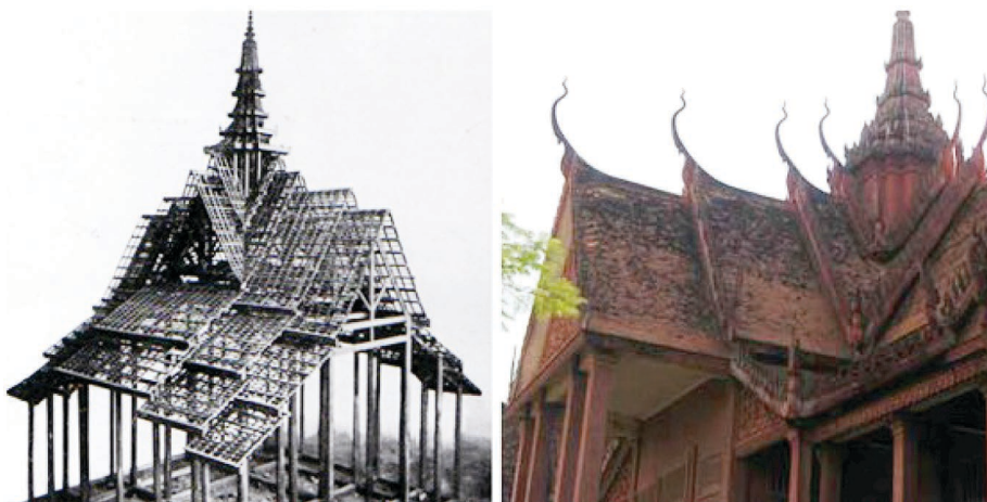
Fig. 12 Left: a photograph of a scale model detailing the internal roof structure of the School of Cambodian Art in Phnom Penh (1921). Right: the roof over the main entrance to the National Museum of Cambodia (2008).
