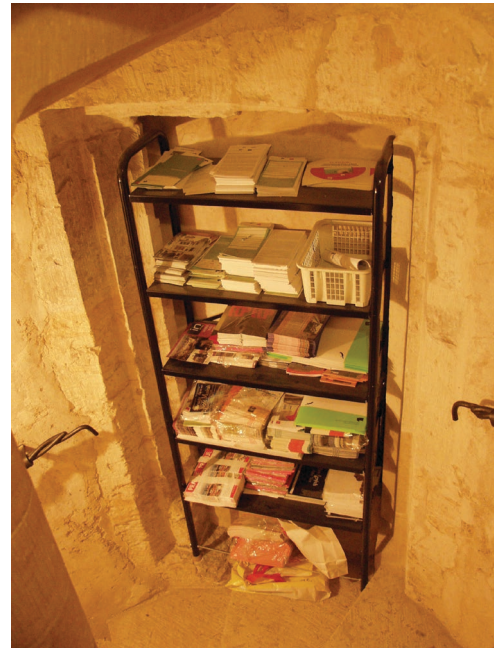
Fig. 29b Rectangular portal between ground floor and first floor, the same as fig. 28 and 29c (2010).
