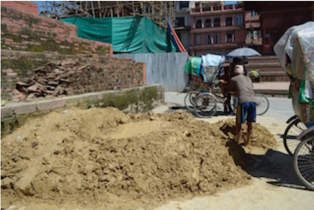
Figure 4.3: Workers preparing the mortar for repairing the roof and the temples in the Durbar Square. (Source: Author/ 2014)
