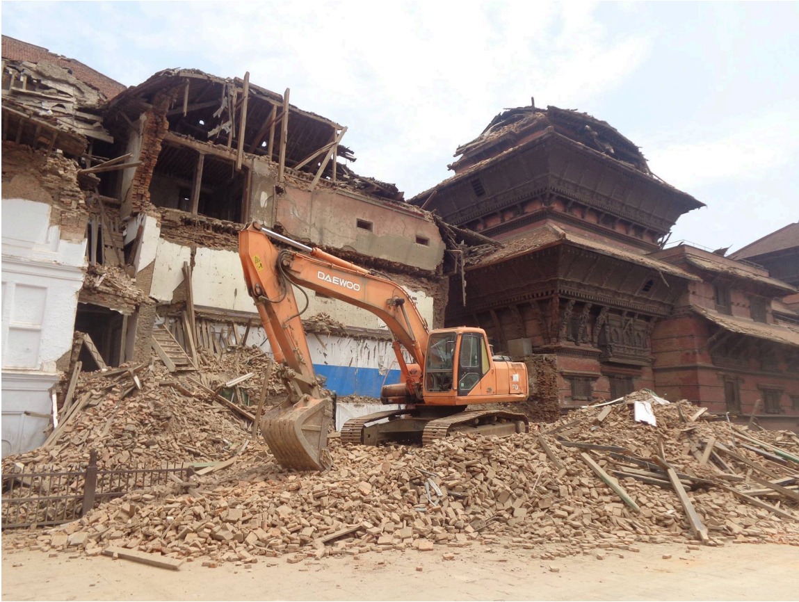
Figure 7.2: Heavy machinery being used after the earthquake to clear the rubbles of the ancient building in the Hanumandhoka Durbar Square. Many experts have criticized this kind of act but it continued. (Source: Kai Weise/2015)
