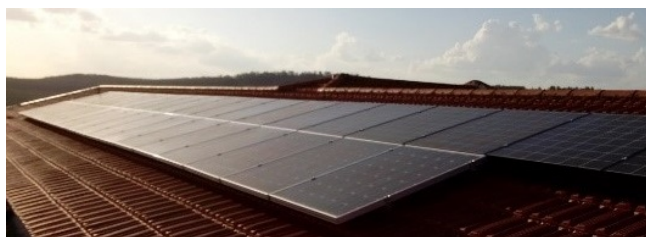
Figure 2. Roof mounted PV system.
