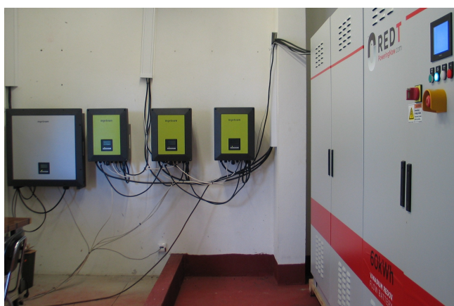
Figure 3. VRFB (right) and the inverters (left).
