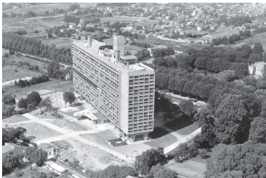
Fig. 2: Marseille Housing Block
