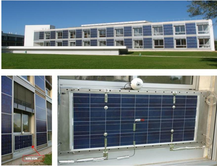
Fig. 5.1. Solar XXI building (top), Prototype installed on the Solar XXI main facade (bottom) [37]
