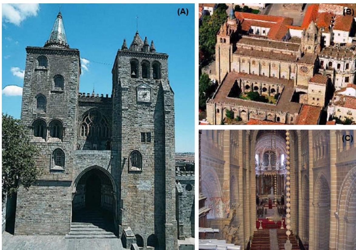
Figure II-3. General view of the façade (A), lateral (B) and indoor of Évora Cathedral, Évora, Portugal.
