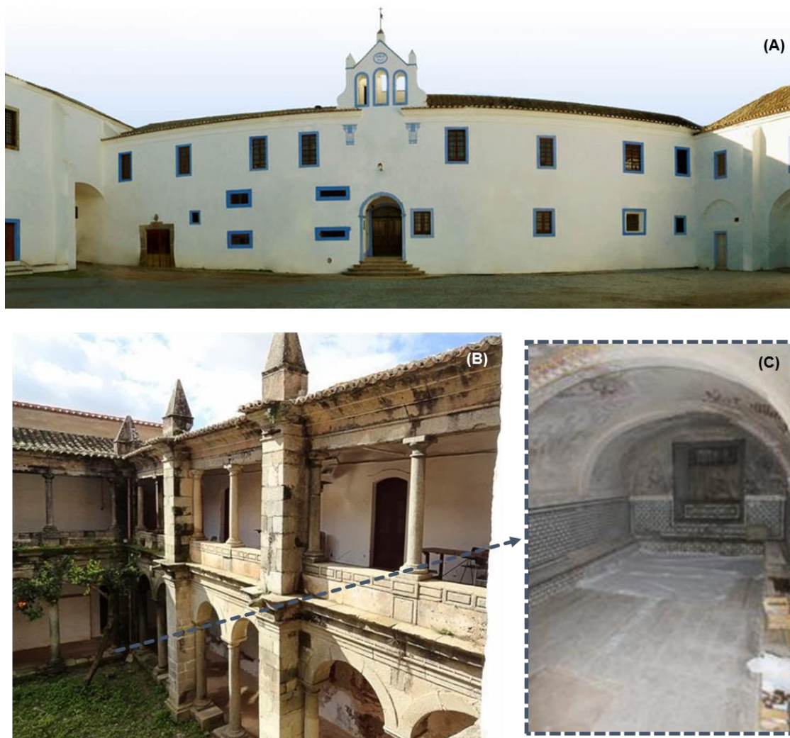
Figure II-2. General view of Nossa Senhora da Saudação Convent, Montemor-o-Novo, Portugal (A), cloister (B) and Low Choir of the Convent (C).
