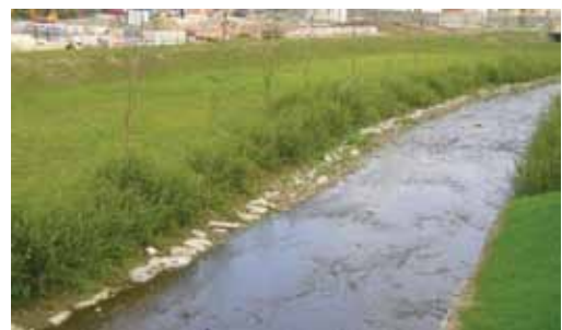
Figure 4.5.4.5 Brush mattress in an urban stretch. Artia stream in Irún (Guipúzcoa, Spain) (Photo: Paola Sangalli).
