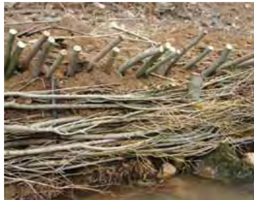
Figure 4.5.3.4 Wattle fence reinforced with live stakes. Tuéjar river in Valencia, Spain (Photo: Antoni Bonafont).
