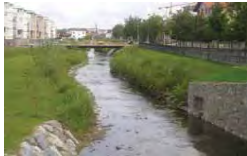
Figure 4.5.5.5 View of the rehabilitated Artia stream in Irún (Guipúzcoa, Spain) (Photo: Paola Sangalli).
