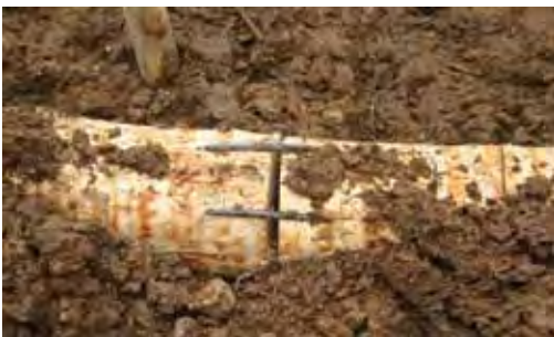
Figure 4.5.5.2 Joining logs together with corrugated steel u-nails (Photo: Antoni Bonafont).
