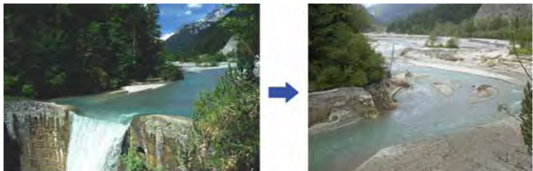
Figure 5.5.7 Removal of sediment-retaining dams, taking the Hornbach as an example.
