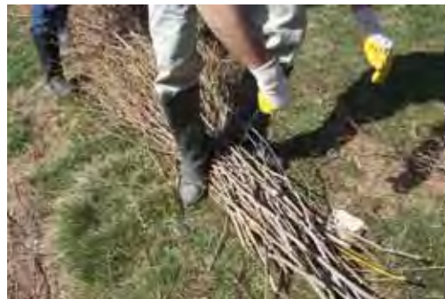
Figure 4.5.1.3 Building a fascine from willow twigs (Photo: J. P. Fernandes).
