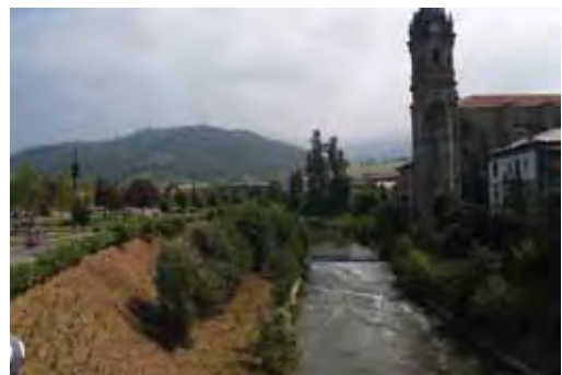
Figure 4.5.2.5 Reinforced slope with live stakes (Photo: P. Barraqueta).
