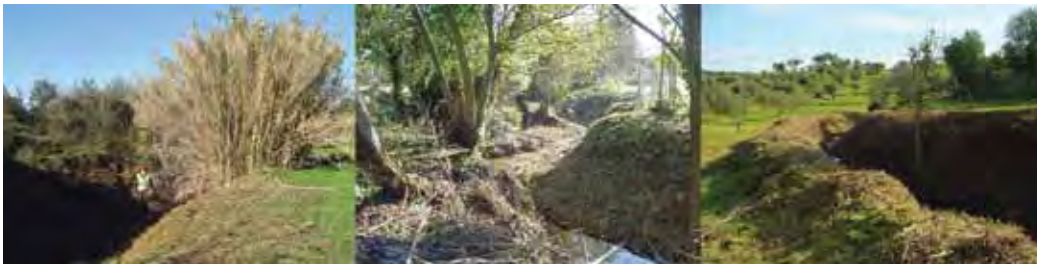
Figure 5.2.3 Examples of contracted restoration work carried out along the two reaches (Gandum Stream and Almansor River) (Photo: F. Pais).
