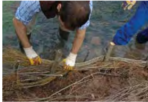
Figure 4.5.3.3 Weaving live willow withies around living stakes. Tuéjar River in Valencia, Spain (Photo: Ana Mendes).
