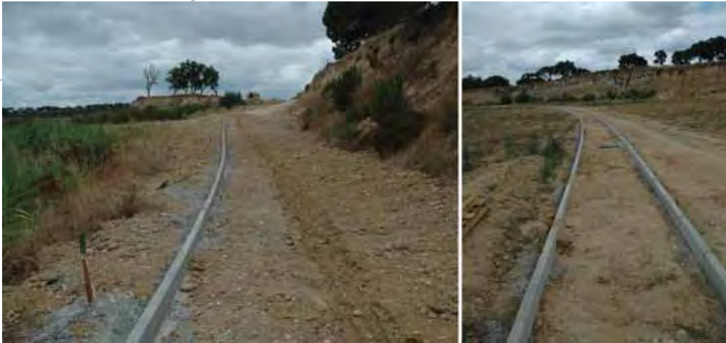
Figure 5.1.8 General aspect of the kerbs used for the interpretation trails (Photo: Ana Mendes).
