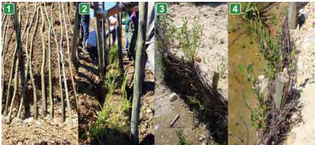
Figure 5.1.25 Woven fences (1); fascines (2); brush mattress (3) and bio roll (4) (Photos: Regina Carriço, 1 and 2, and André Fabião, 2 and 3).
