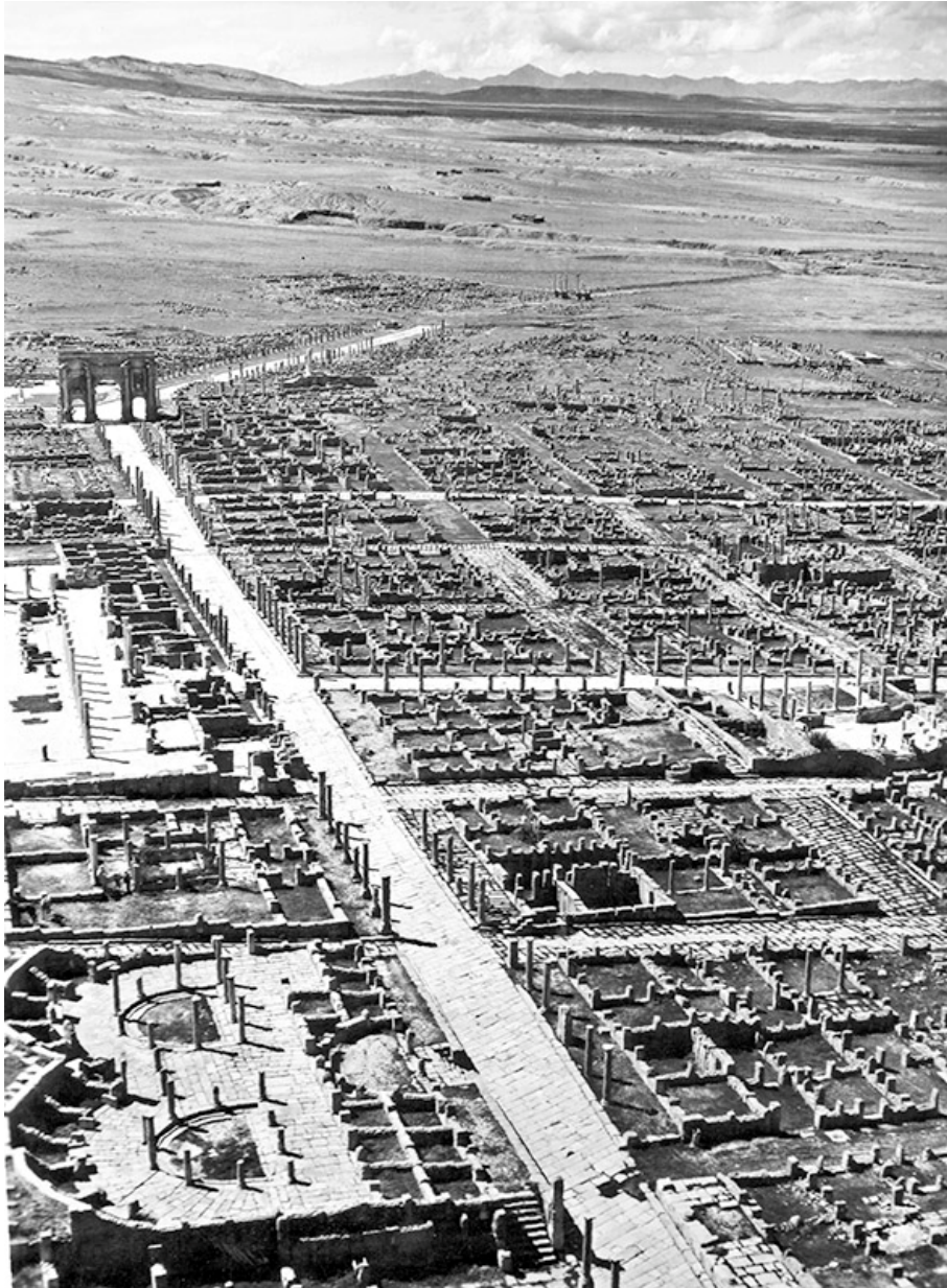
Fig. 5.6 Ruins of the Roman city of Timgade in now Algeria (photo by A. Crosnier). Note the street network designed for near optimal flow access, very close to optimized constructal design.
