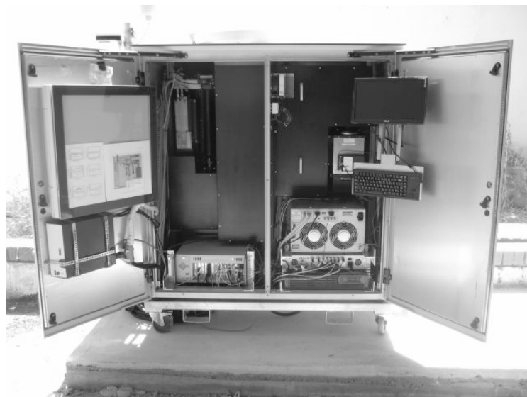
Fig. 9a. View of the open LIDAR System set up at Évora.
