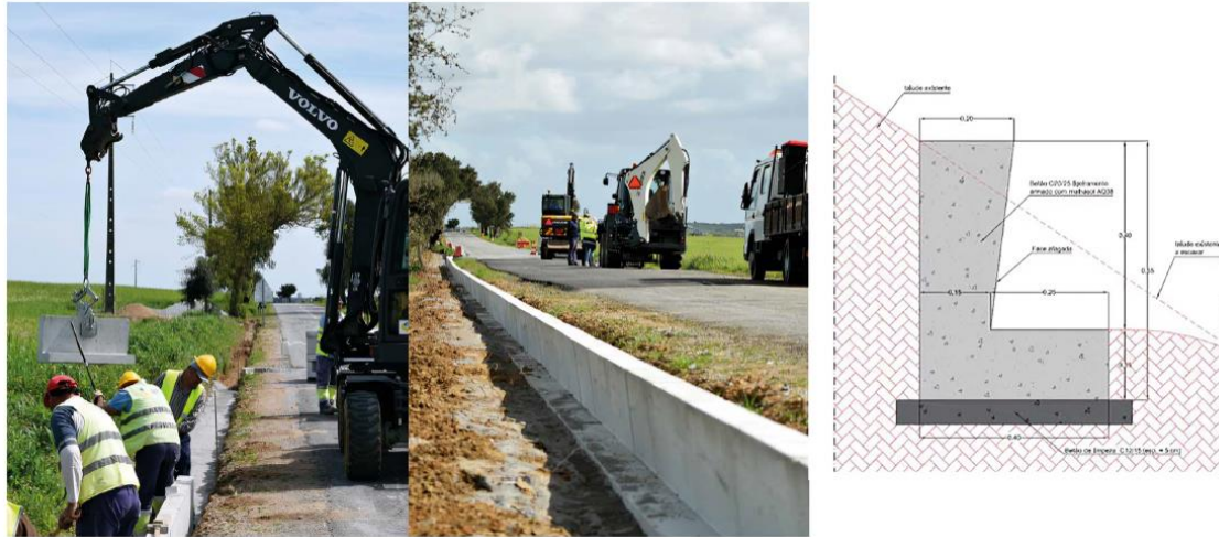
Figure S4.1. Installation of permanent concrete drift fences as well as a cross-cut of the “L” shaped piece with a slight inclination of the wall towards the outer side of the road (source: Garcia et al., 2021).
