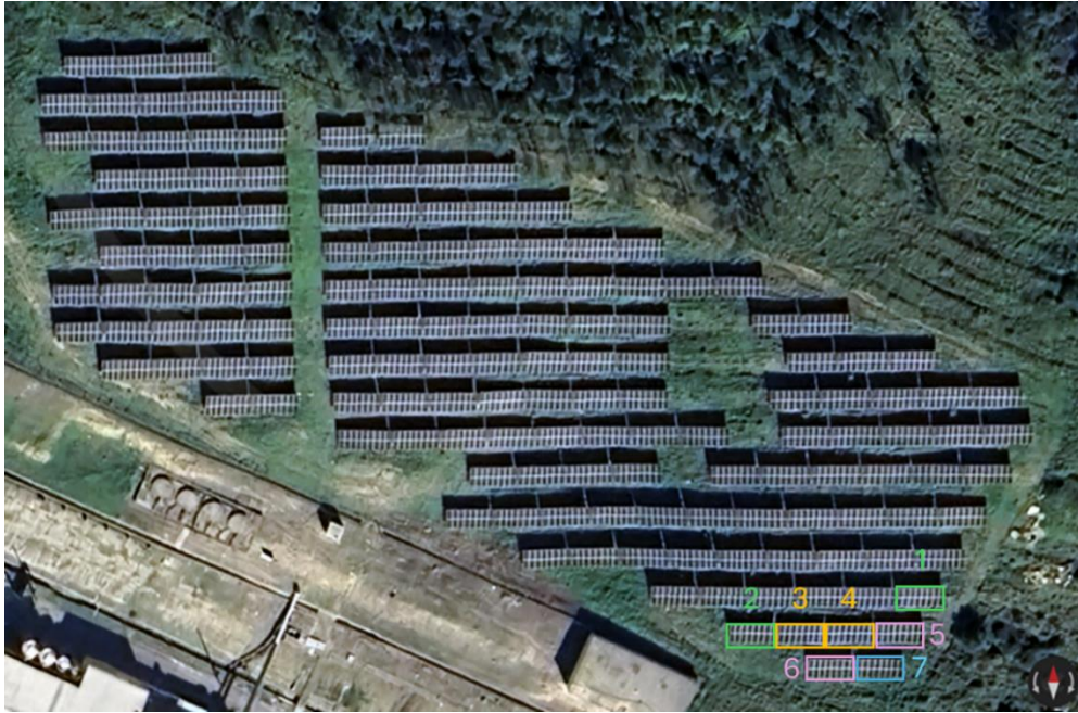
Fig. 6.7 - Aerial view of the photovoltaic powerplant (1-7: strings considered in the work).
