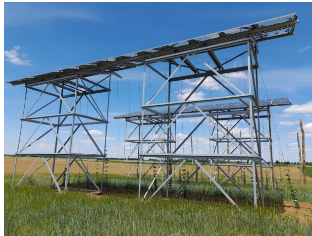
Figure 2.9: Agrivoltaic structure for hop growth [84].
