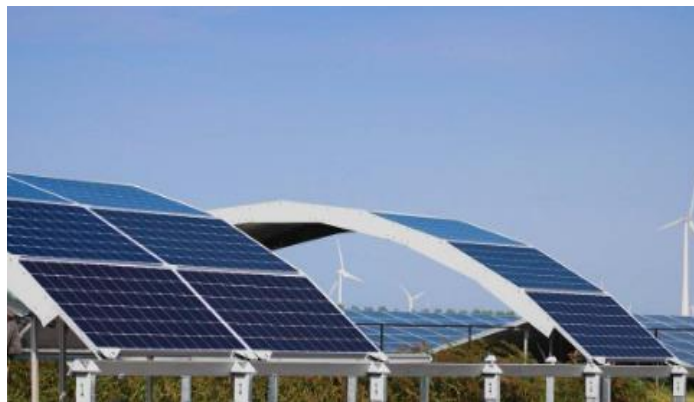
Figure 2.10: Arc-shaped PV modules developed by Goldbeck Solar [86].
