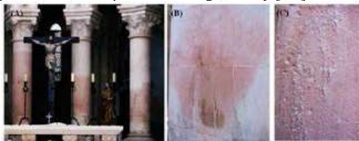
Figure 1: (A) distinct phenomenon observed at the altar of the monastery church; (B) pink colored biofilms on the walls; (C) evidence of the presence of salts on the walls.
