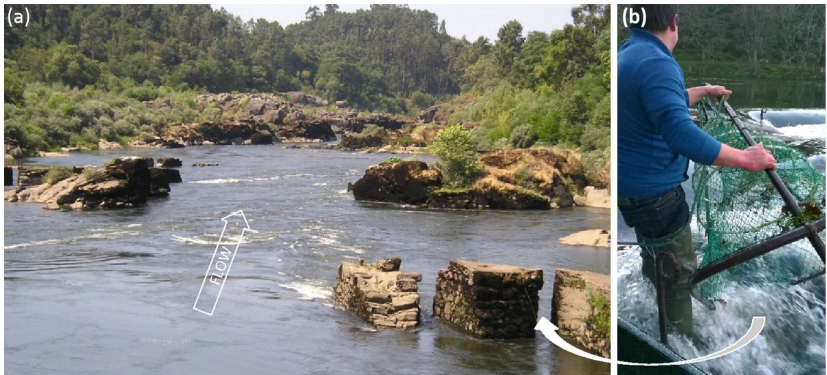
Fig. 4 Fishing weir ( pesqueira ) at river Minho used to target anadromous species in Northwestern Iberian Peninsula rivers ( a Image: Bernardo Quintella). Some weirs have vertical slots
