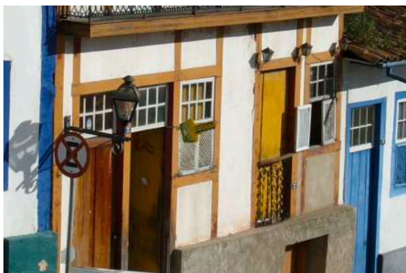
Figure 89 Example of the openings of a house, with their painted beams, sills, and jambs. It is possible to observe the elongated beans and jambs, and the use of the same bean for different openings. Source: Martins [2010] 308 .
