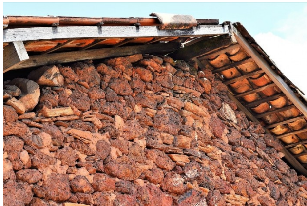
Figure 79 Wall made of pedra e barro and without the wall plaster in a house of Ouro Preto. Photo by Elio Moroni Filho. Source: Moroni Filho [2020]. 296
