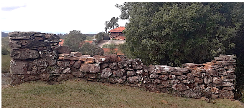
Figure 78 Wall made of pedra seca (dry-stone masonry) in Ouro Preto. Photo: author, 2018.
