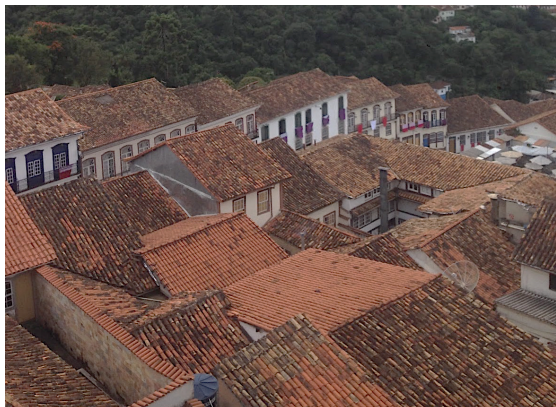
Figure 90 Roofs in Ouro Preto. Source: author.
