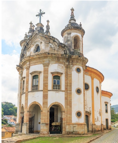
Figure 48 Photo of the church of Nossa Senhora do Rosário of Ouro Preto. Photo by Rodrigo Argenton. Source: Wikipedia [2017]. 232
