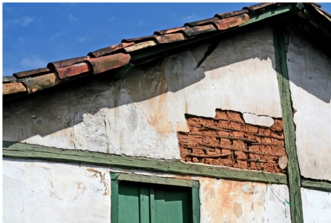
Figure 85 Pau-a-pique used to seal the wood structure of a house in Ouro Preto. Source: Machado [2009] 303 .
