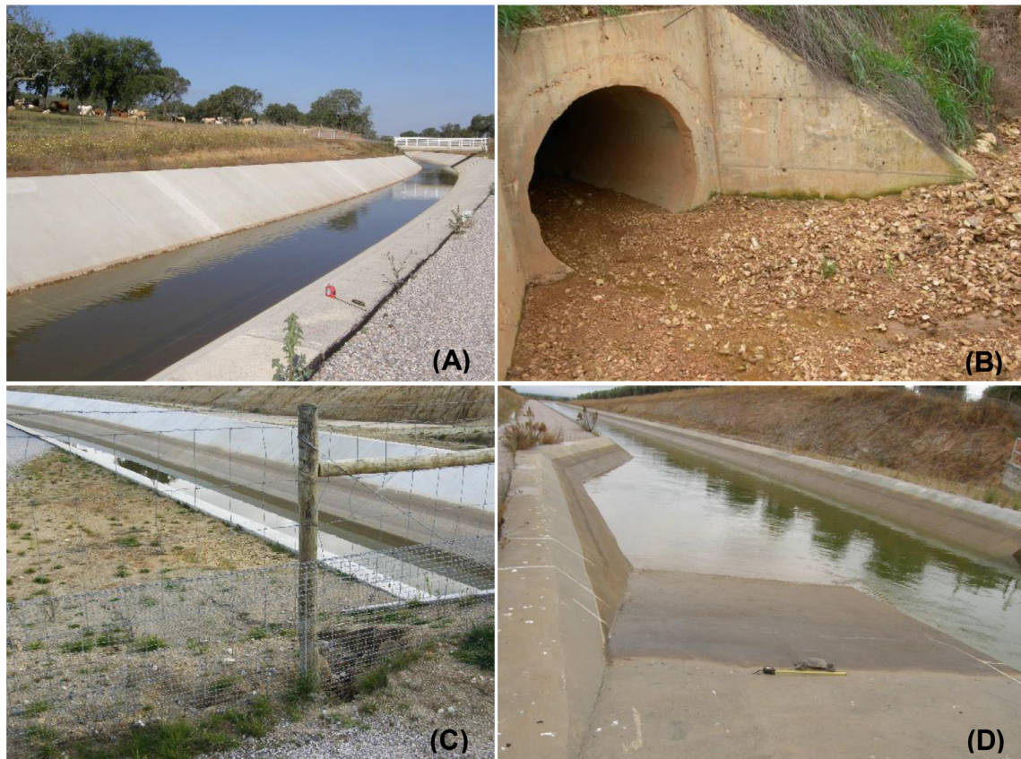
Fig. 2. Overpass (A), culvert (B), fence (C) and wildlife escape ramp (D) at the Alqueva irrigation canals.
