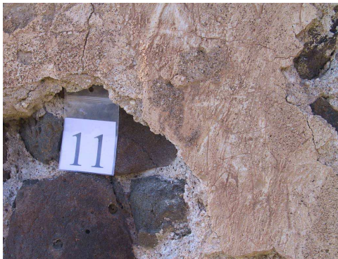
Fig. 18 - FOG-M11 sample – external finish coating
