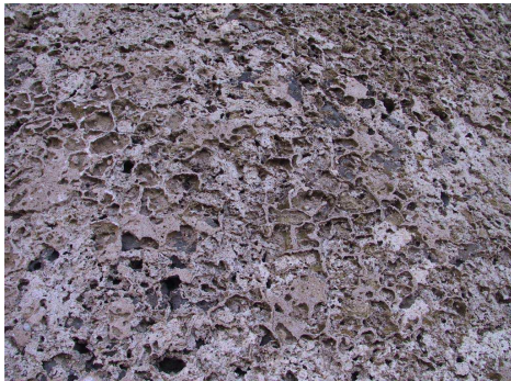
Fig. 14 – Torre di Foghe, tafones like-honeycomb in the exposed NO surface of the tower
