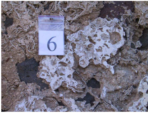
Fig. 17 - FOG-M6 sample – Plaster
