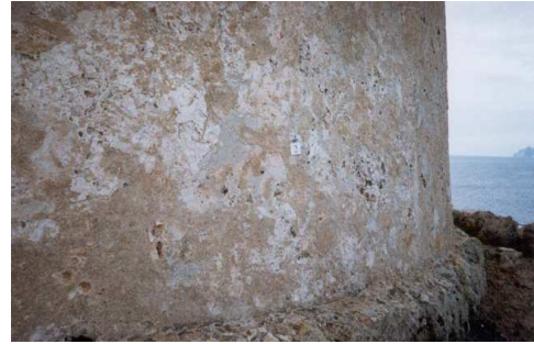
Fig. 3 - Northern side of the tower: wall covering partially restored
