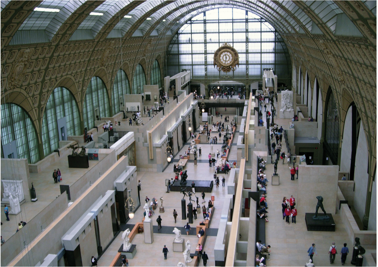
Figure 2 | View of the nave of the Gare d'Orsay converted into the Musée d'Orsay. Source: Wikimedia Commons (accessed 2 April 2020).
