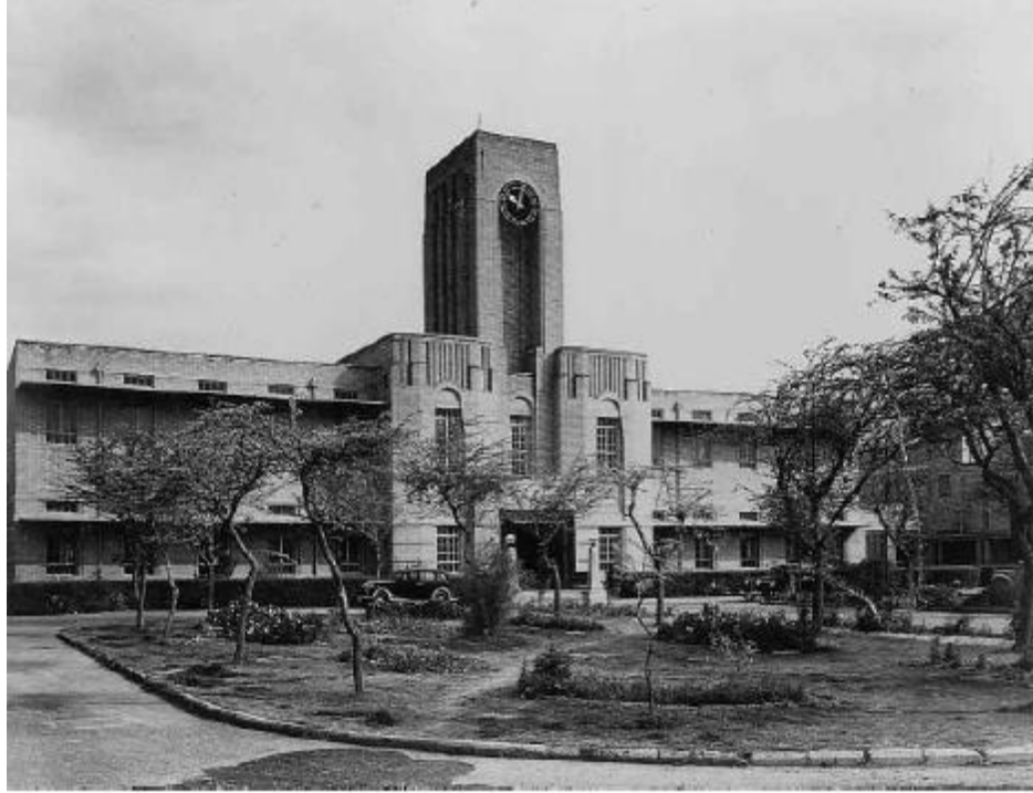
Figure 3 : Abadan Technical Institute, Abadan. (Photo: Wilson Mason and Partners). 30
