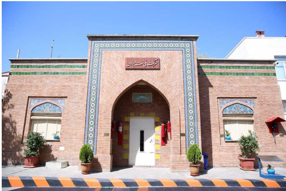
Figure 8 : The main building of Darvazeh Dolat Gas Sation Museum, 2020. 36
