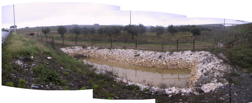
Fig. 1. Infiltration pond at A2 road, Borba, Portugal
