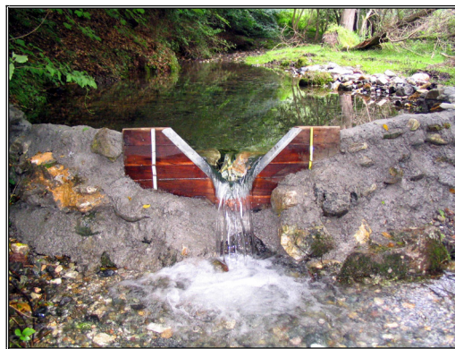
Fig 2. Weir of natural material-spring Ljubivoda
