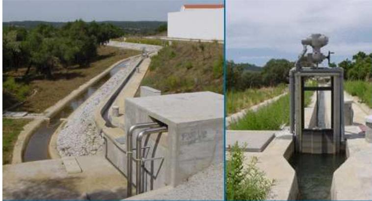
FIGURE 1. Overall view of the pilot channel and detail of one gate
