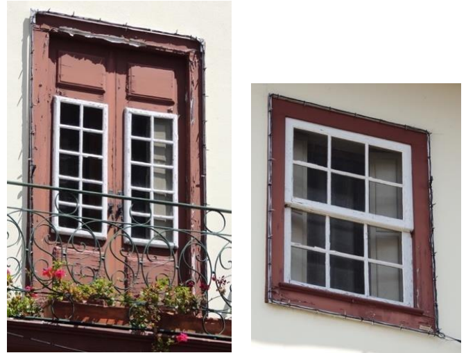
Figure 3: Caption of frames of south façade of Pousada Nossa Senhora das Oliveiras. New double glazing windows and doors painted with two different colours. Luísa Ghignatti, 2015.
